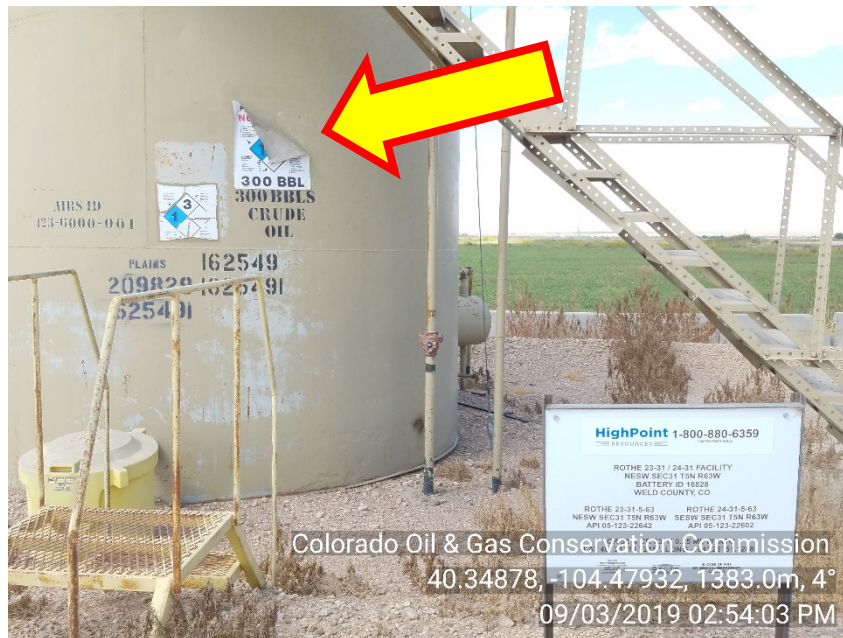
Photo #3 Rothe 24-31, 23-31 Battery Shut-down | Inactive NFPA Label peeling, NOT legible
