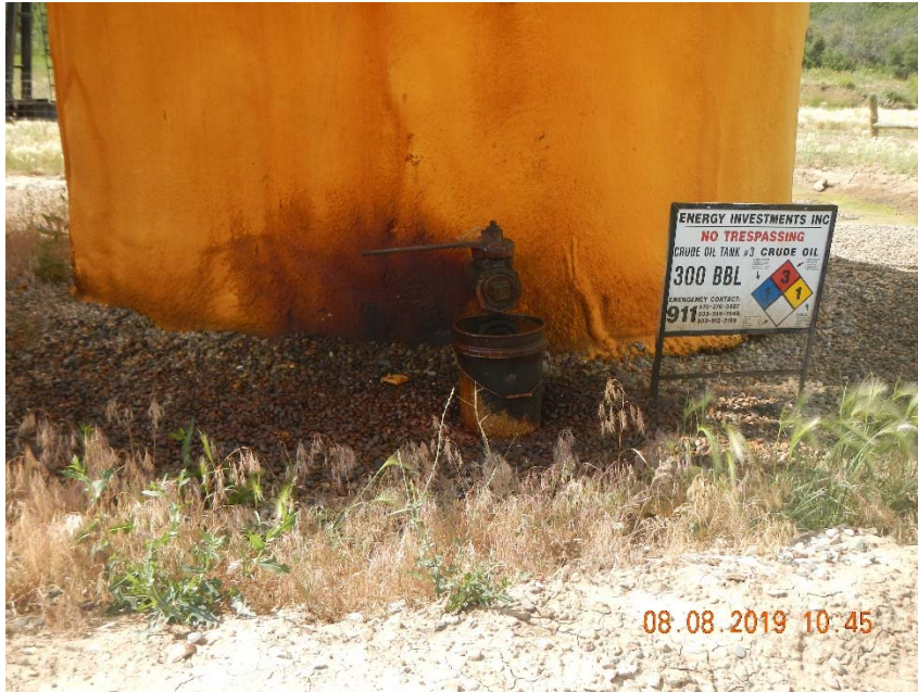
Photo 5. Stained soil with overflowing bucket at tank base.
