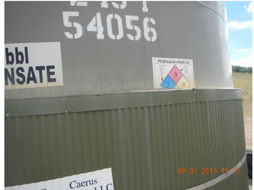
**400 bbl tank has label for condensate and for petroleum crude oil. NFPA hazards have conflicting levels.**
