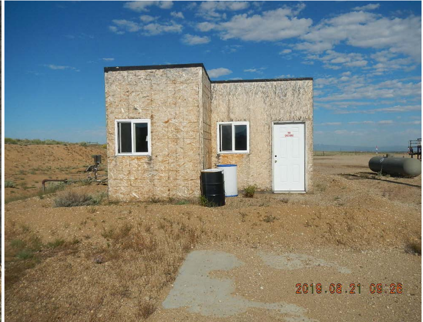
Chemical storage (antifreeze) in inadequate secondary containment, vegetation growth near equipment building.
