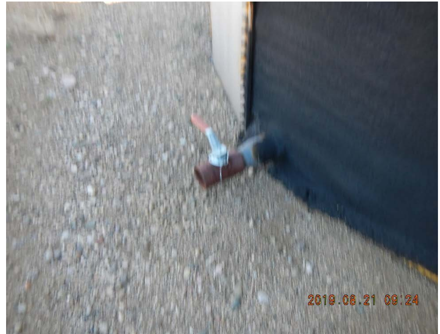
Valve with handle not blind plugged. Note: There was evidence of livestock accessing Facility.
