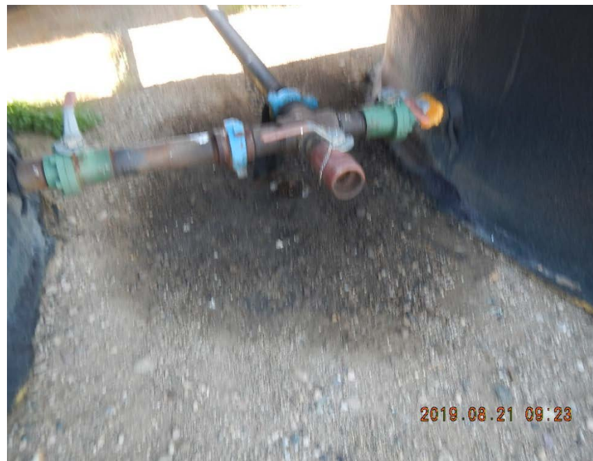
Tank 0030, staining beneath hammer unions.
