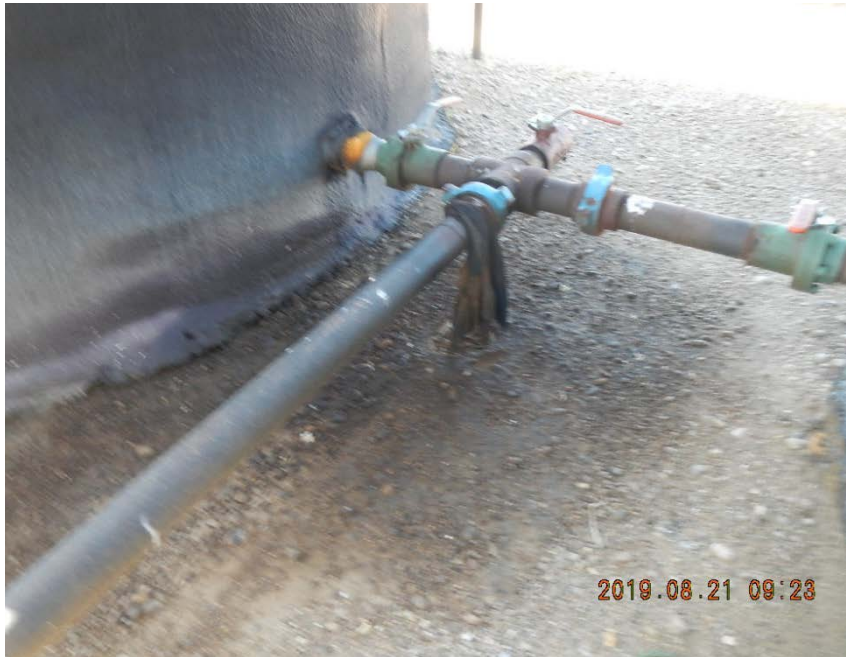
Tank 0030, staining beneath hammer unions.
