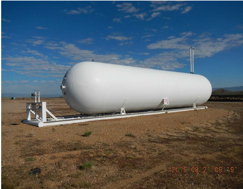
Propane tank not labeled or placard.
