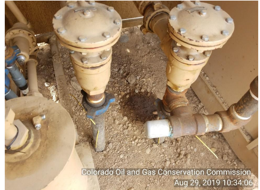
Photo 4 stained soil inside separator house and mechanical issue.
