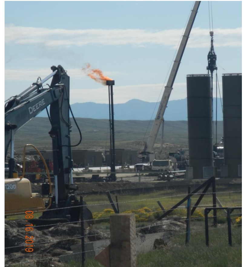
Photo#2: Flare did not seem to be burning efficiently.
