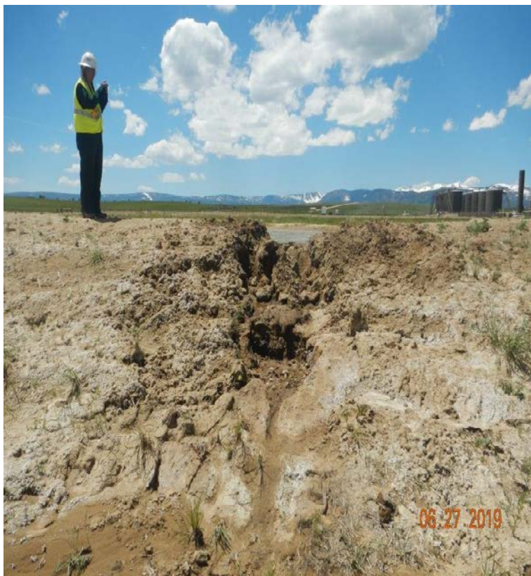
Photo#5: Breach at reservoir berm 6/27/19.
