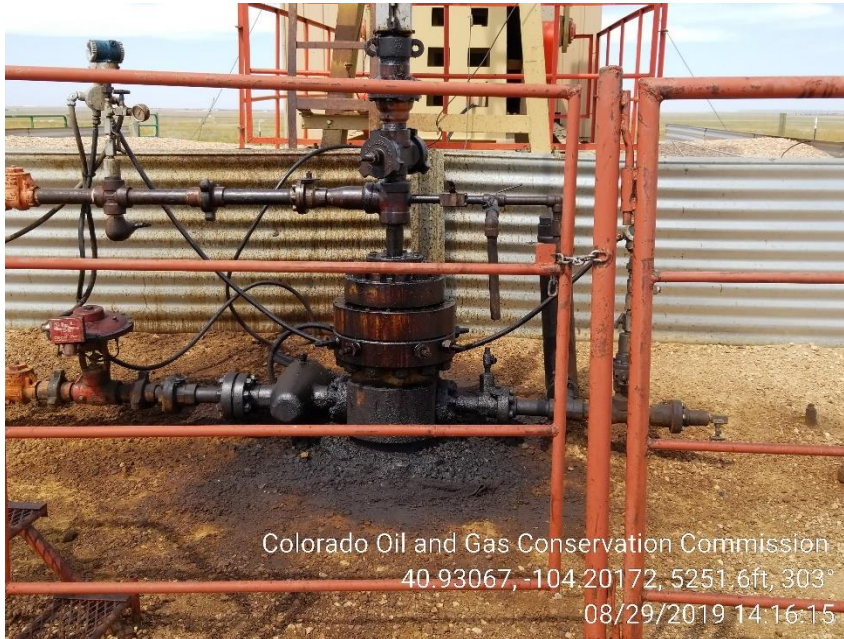
Photo 1 – Mechanical Conditions – Wellhead appears to be leaking onto the ground,
