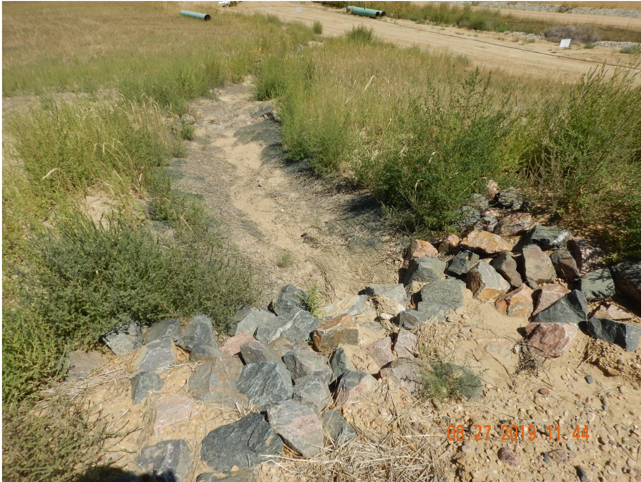
Photo 1. Photo taken of the northeast battery location, facing North. BMP maintenance is required. Also, the installed stormwater BMPs do not appear to be installed with good engineering practices, as the check dams are spaced too far apart to slow the velocity of stormwater runoff. Photo also illustrates unmanaged weeds.
