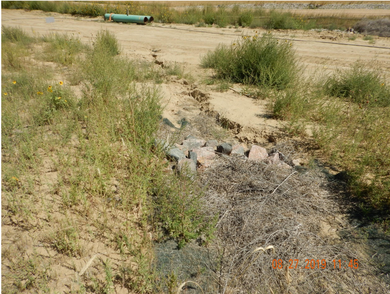
Photo 2. Photo taken at the end of the stabilized channel, facing East. Photo illustrates erosion and BMP maintenance is required.
