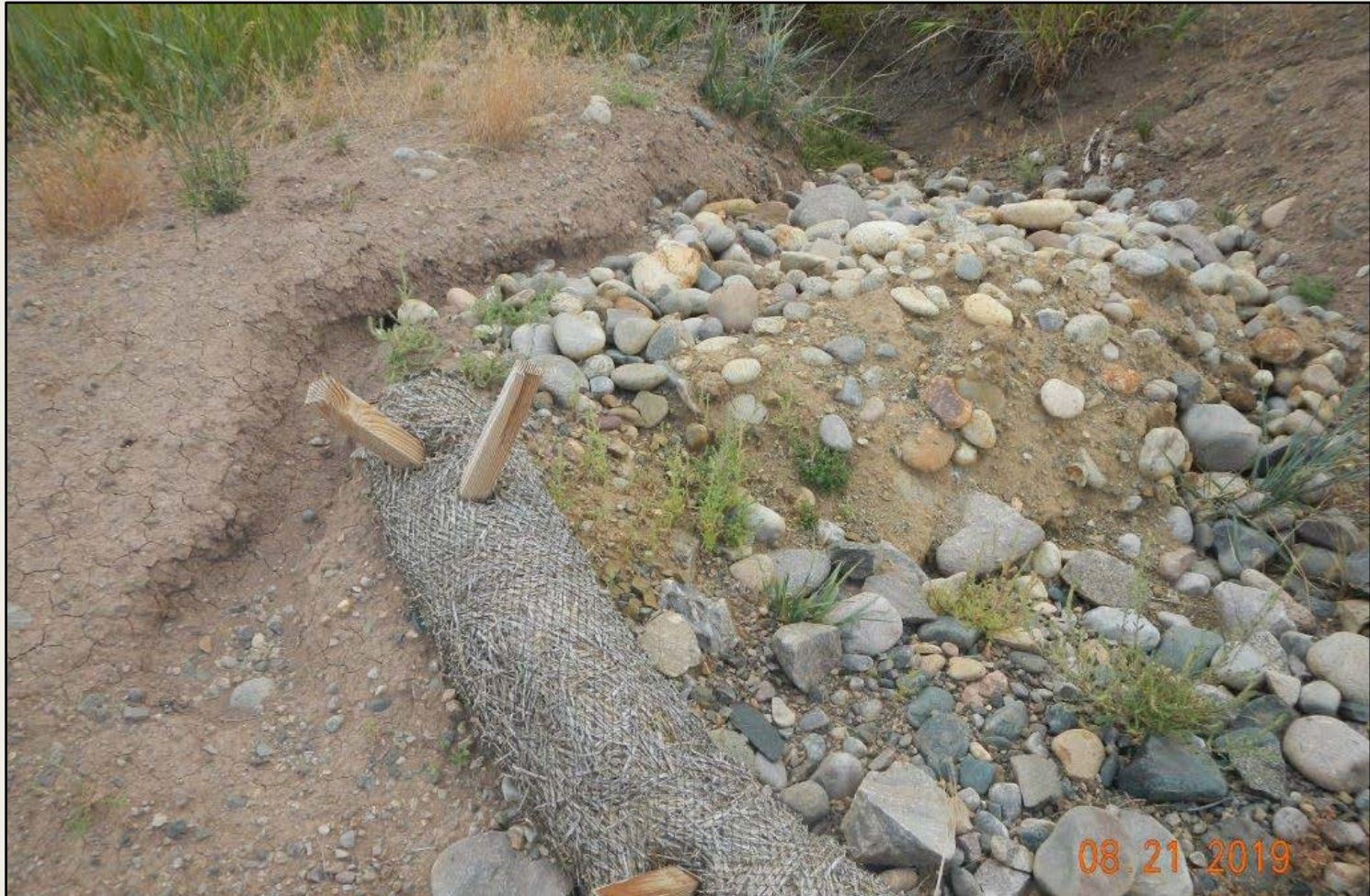
Photo 3. View of area where concentrated run-off exits the well pad and stormwater BMP is failed.
