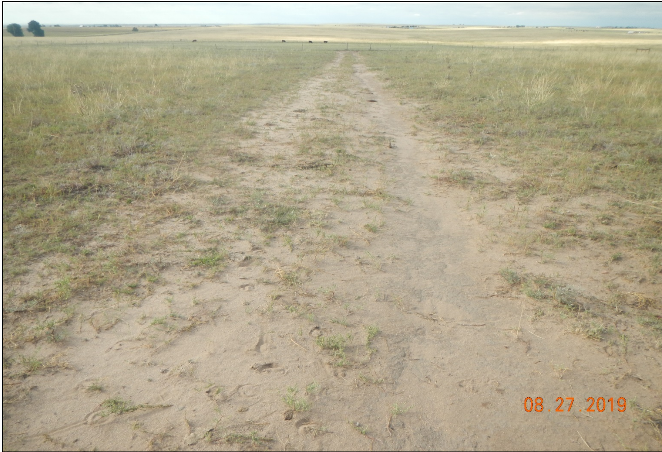
Photo 1. Facing south along the access road. There may be compaction issues along the road preventing revegetation.
