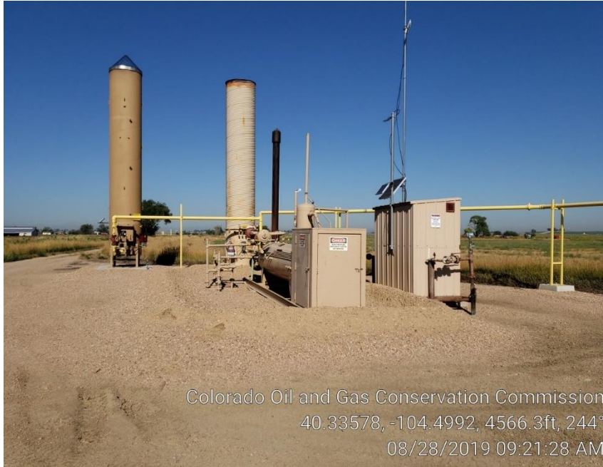
Photo # 3 Separator, ECD's, & Meter Run
