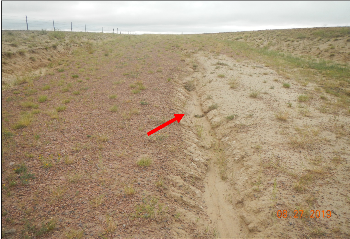
Photo 3. There is an erosion channel along the access road as it ascends the hill.
