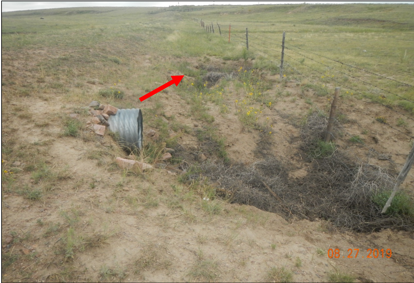
Photo 2. There is no outlet protection at the outlet of the culvert and signs of erosion.
