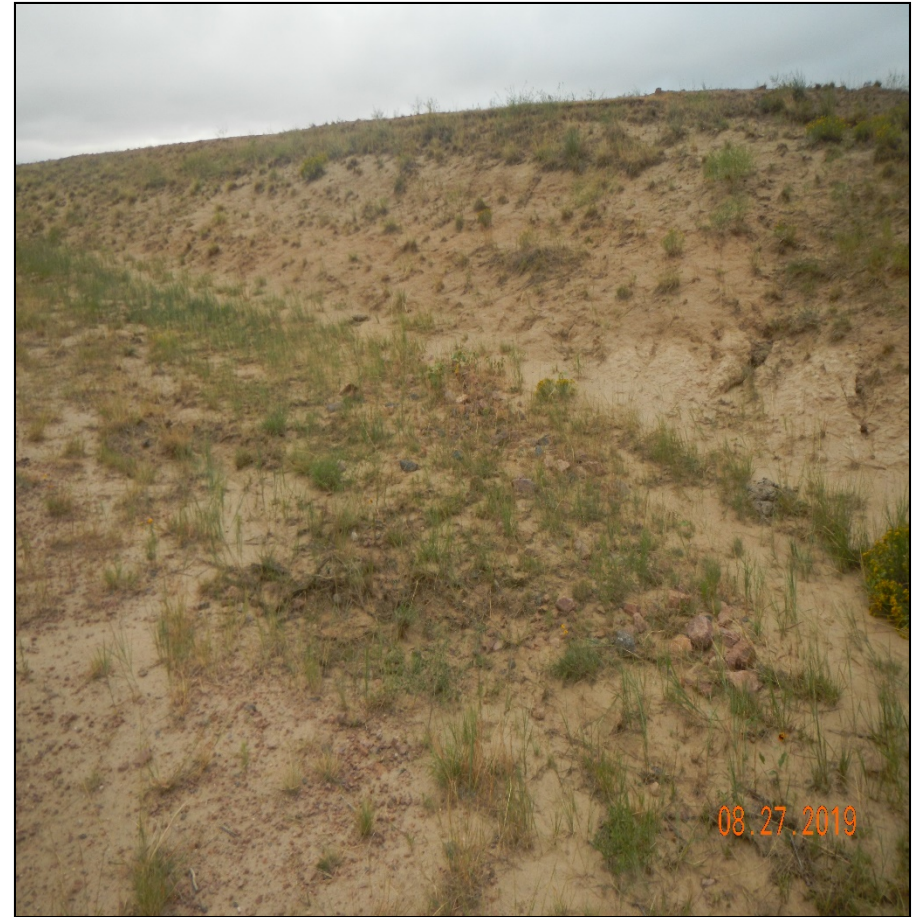
Photo 4. The sides of the access road as the road ascends the hill are not stabilized and no BMP's are present.
