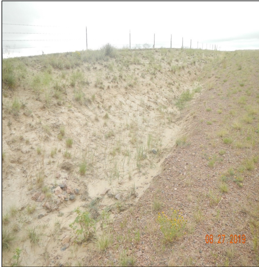
Photo 4. The sides of the access road as the road ascends the hill are not stabilized and no BMP's are present.
