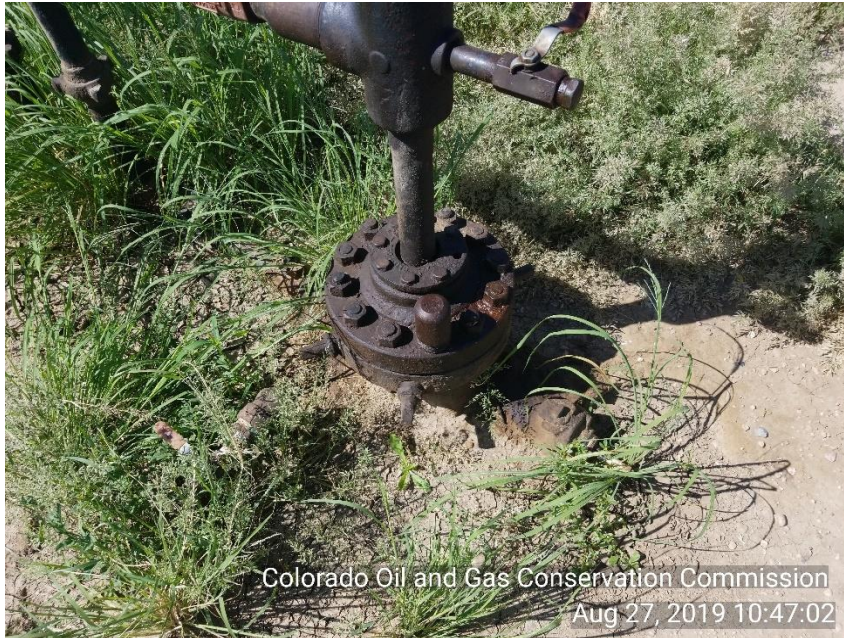
Photo 3 Stained soil around WH. Mechanical issue 1" valve on flow line appears to be leaking.
