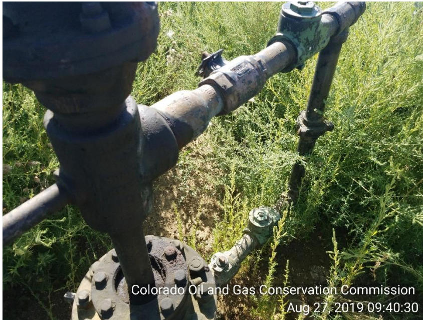
Photo 3 Production flow lines off WH are closed Well is SI.
