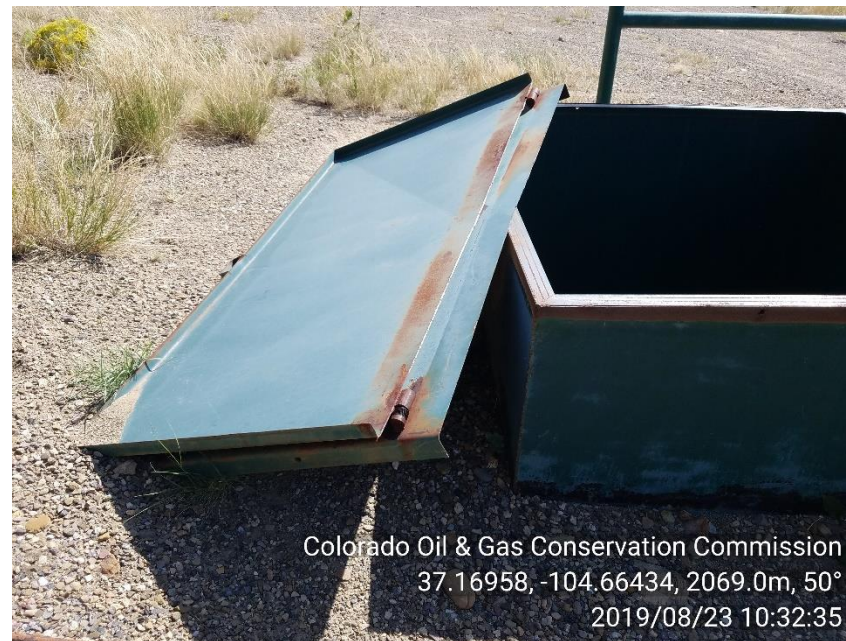
PHOTO 4: UNUSED EQUIPMENT, LID TO UNDERGROUND VALVE BOX IS LEANED TO THE SIDE. REMOVE OR REINSTALL UNUSED EQUIPMENT, COMPLY WITH RULE 603.f. CA DATE 9-23-19
