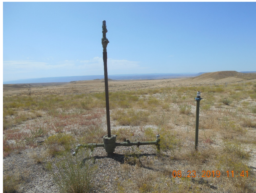
Wellhead Temporarily Abandoned.
