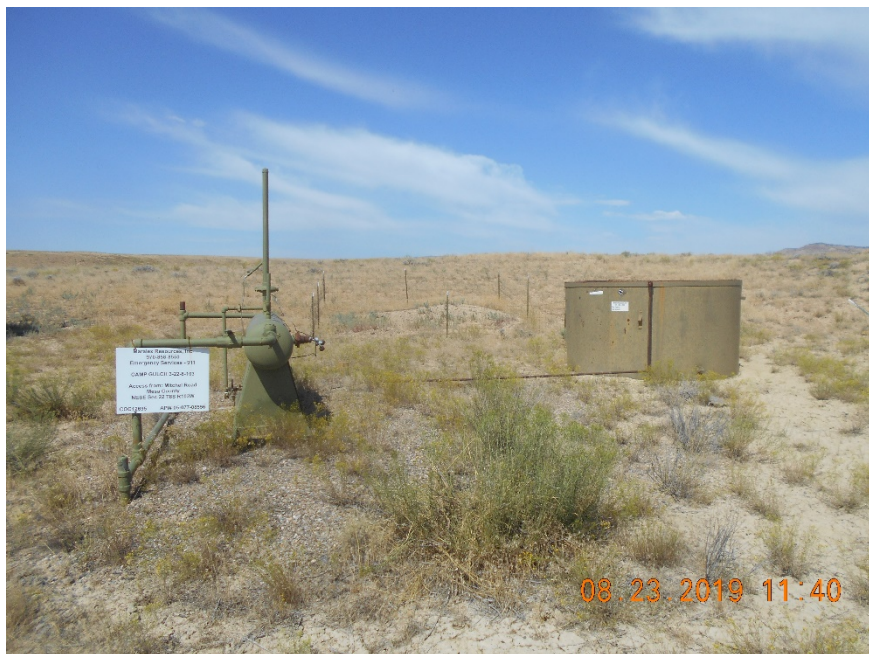
Separator with sign and blowdown tank.
