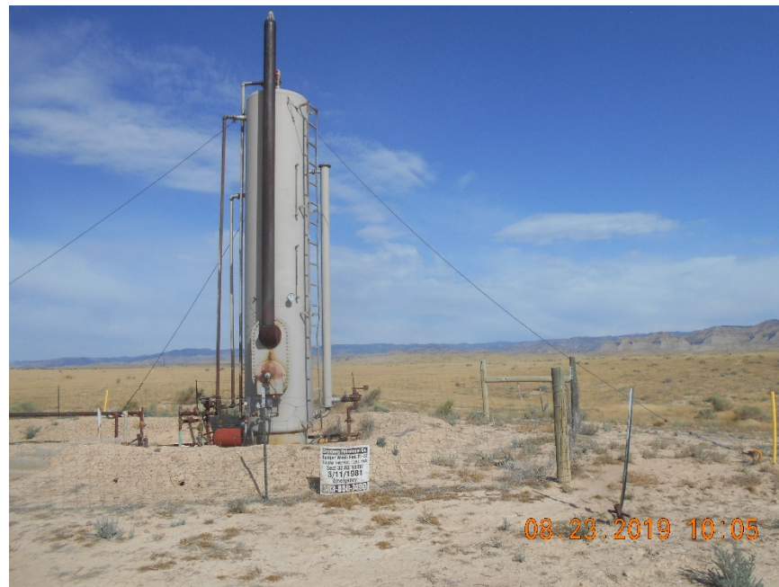
Vertical Separator with sign
