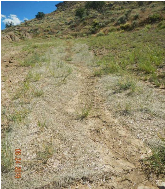
Photo#8: Erosion blanket installed.
