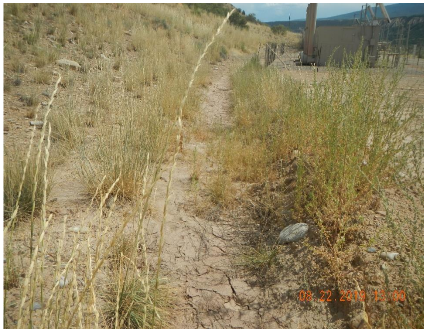
Sediment build up in diversion ditch.
