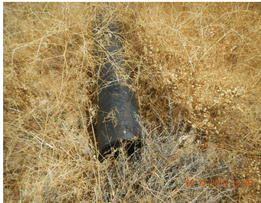
Line comes out on south side road is above ground with an open end.
