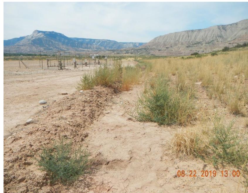
Sediment build up in diversion ditch.
