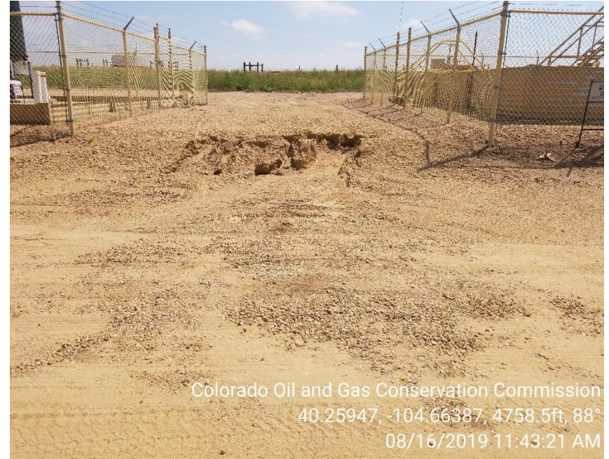
Photo 4 – Erosion occurring between tanks and separators
