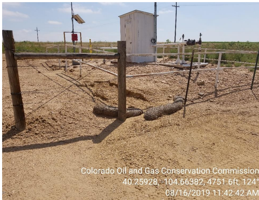
Photo 7 – Erosion occurring south of tanks
