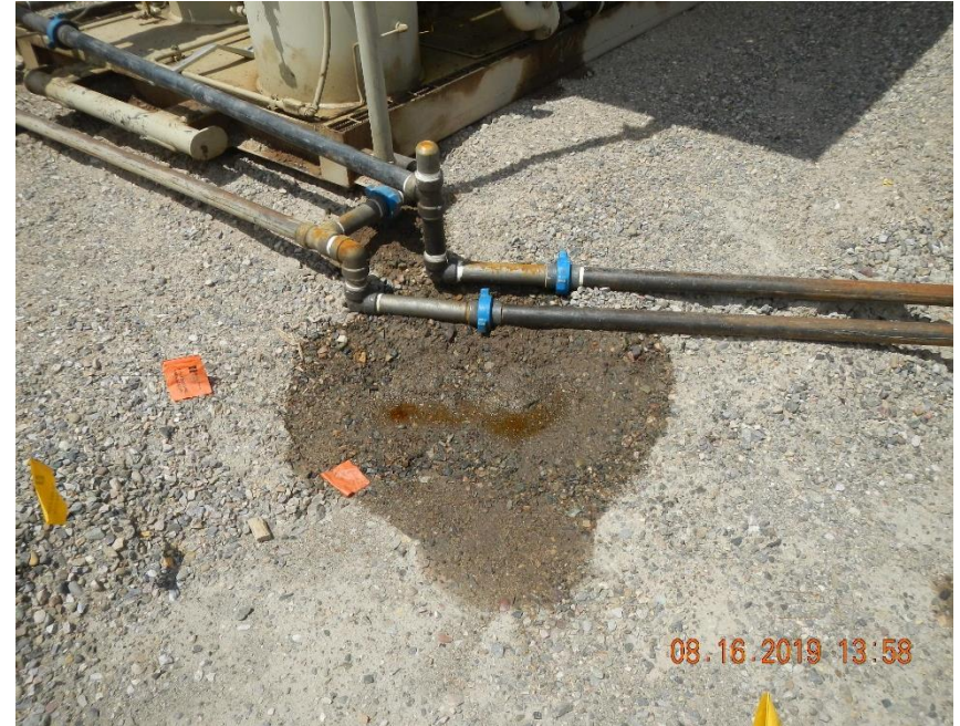
Stained and wet gravel beneath hammer unions on flow lines.
