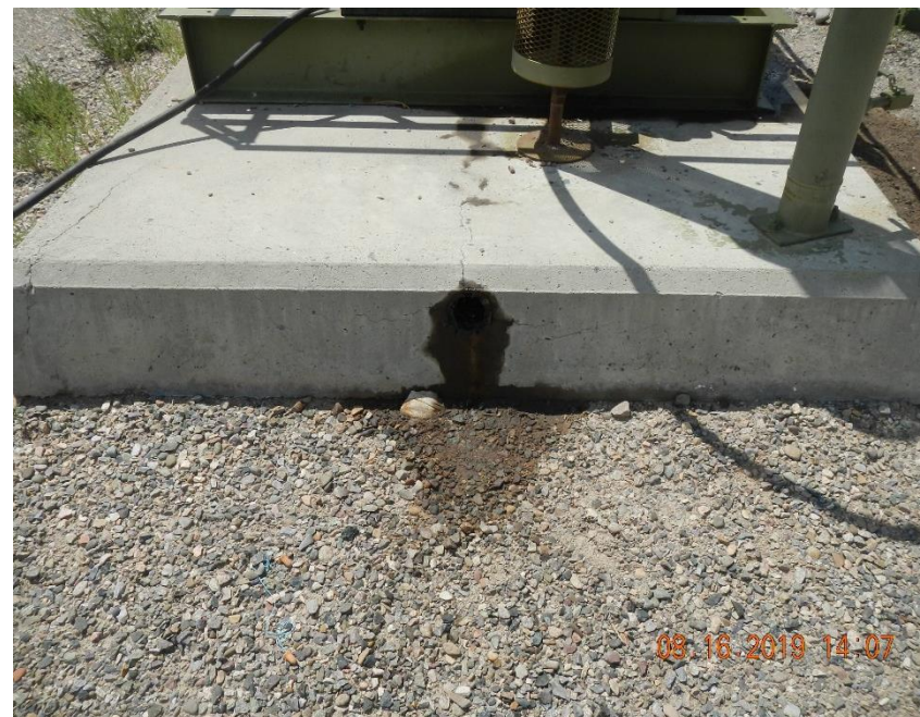
Concrete pad is stained at weep hole and surrounding gravel is stained.
