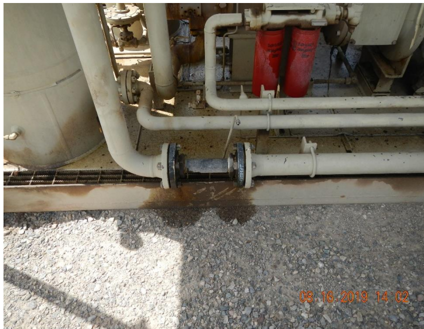
Stained gravel beneath flanges at compressor.
