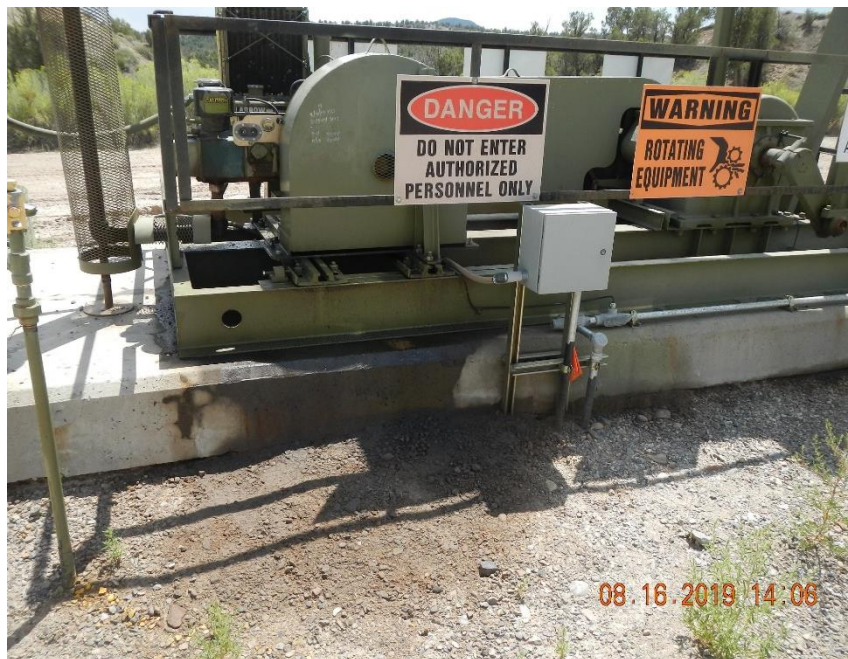
Concrete pad and surrounding gravel is stained and wet.
