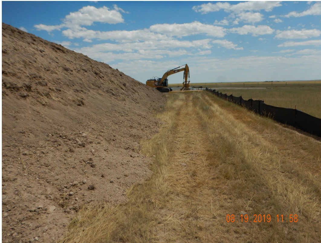
Photo 6. Photo taken from the southern location, facing East. Photo illustrates the topsoil stockpile. Operator plans to reduce the side slopes, seed and straw crimp mulch.
