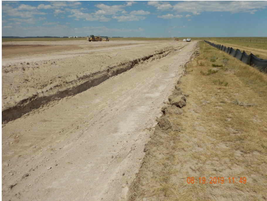
Photo 2. Photo taken from the southeastern location, facing North. Photo illustrates the perimeter BMP (silt fence). Construction operations still underway.
