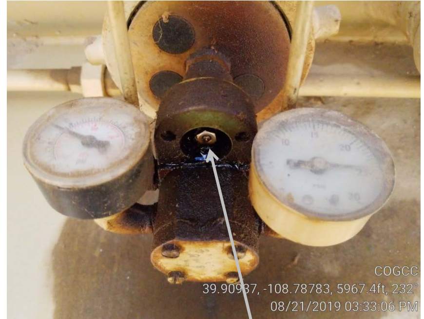
Photo 3. Separator gas leak.
