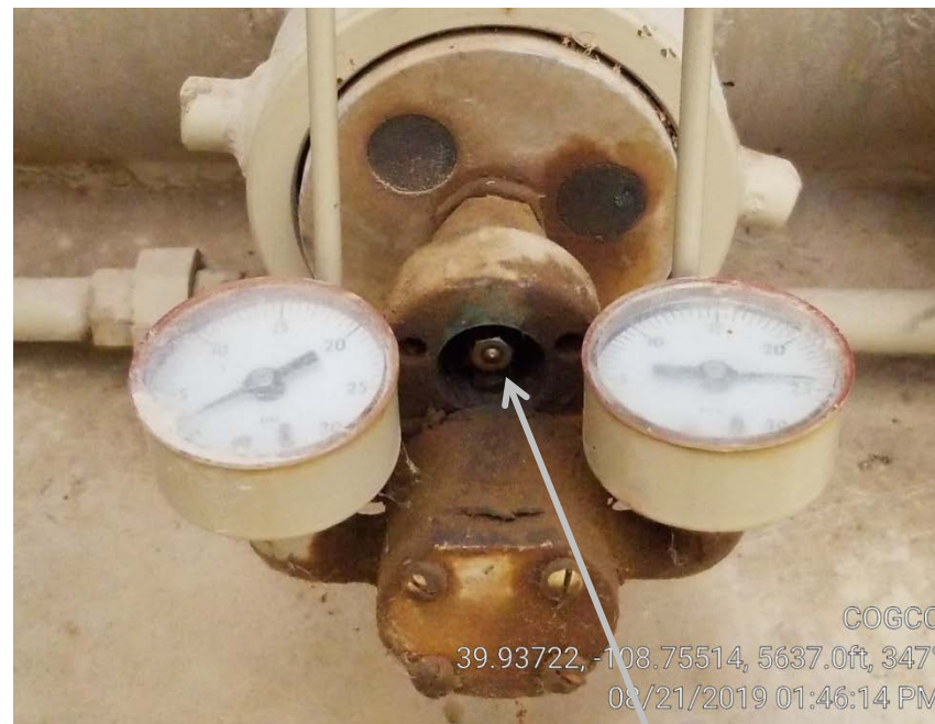
Photo 3. Separator gas leak.
