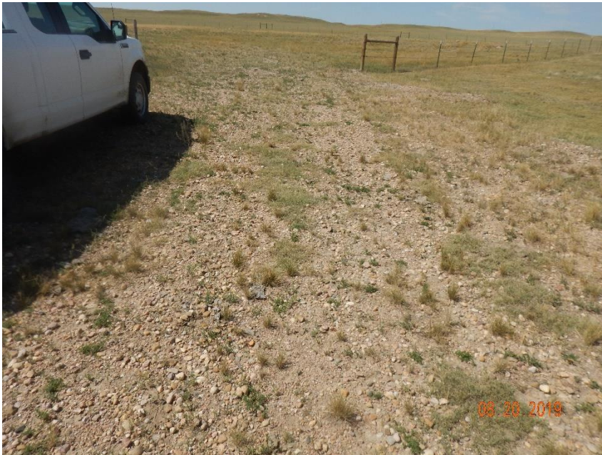
Photo 1: Photo taken from the northeast end of the location, facing southwest. Photo shows gravel/road base remaining on access road. Gravel does not appear to be conducive to reclamation
