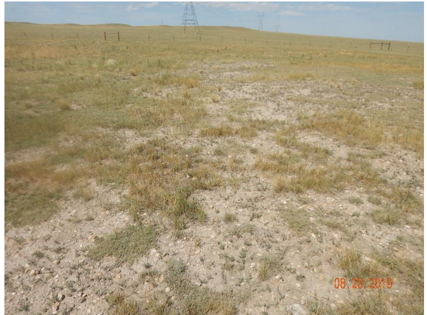
Photo 2: Photo taken from the location, facing southwest. Photo shows gravel/road base remaining on appears to be hindering reclamation.
