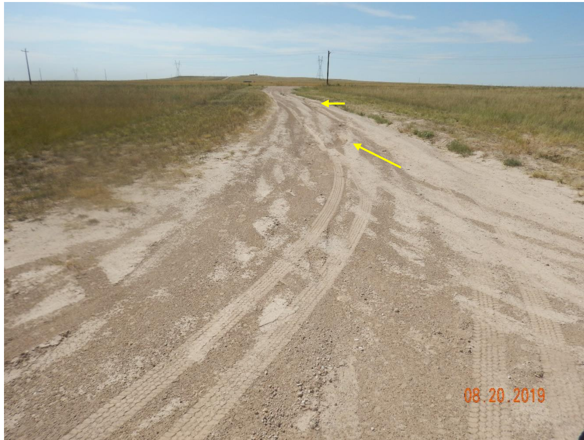
Photo 15: Photo taken from the south end of the location, facing south. Photo shows stormwater erosion degradation on access road.
