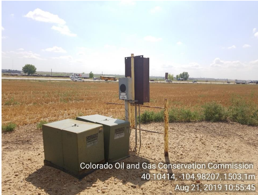
Photo 3 Electrical panel no meter on breaker box
