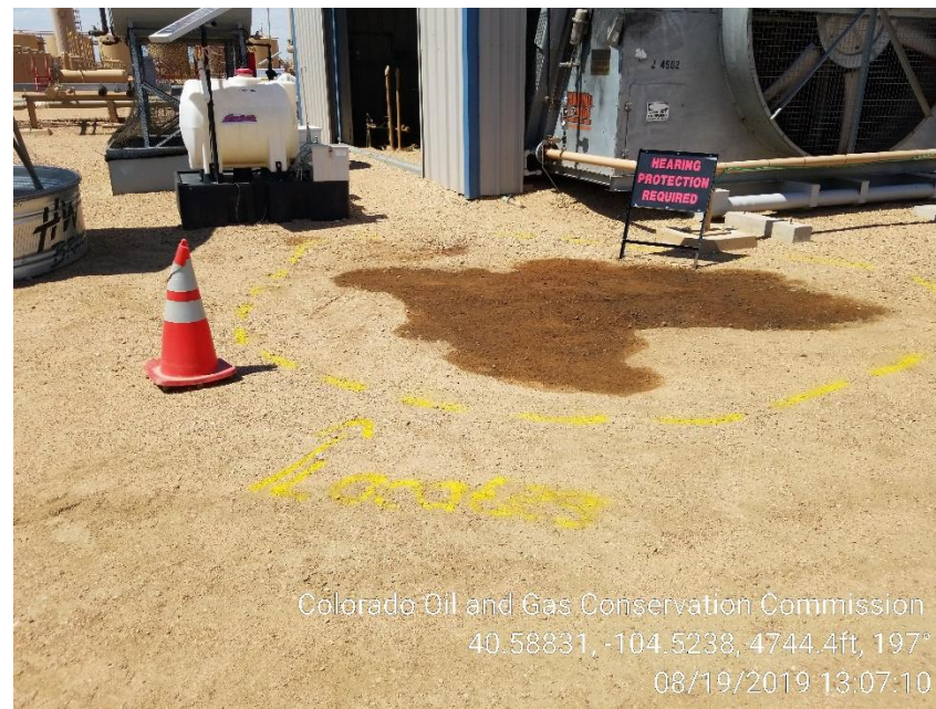
Photo 2 – Stained Soil by the Gas Lift Compressor
