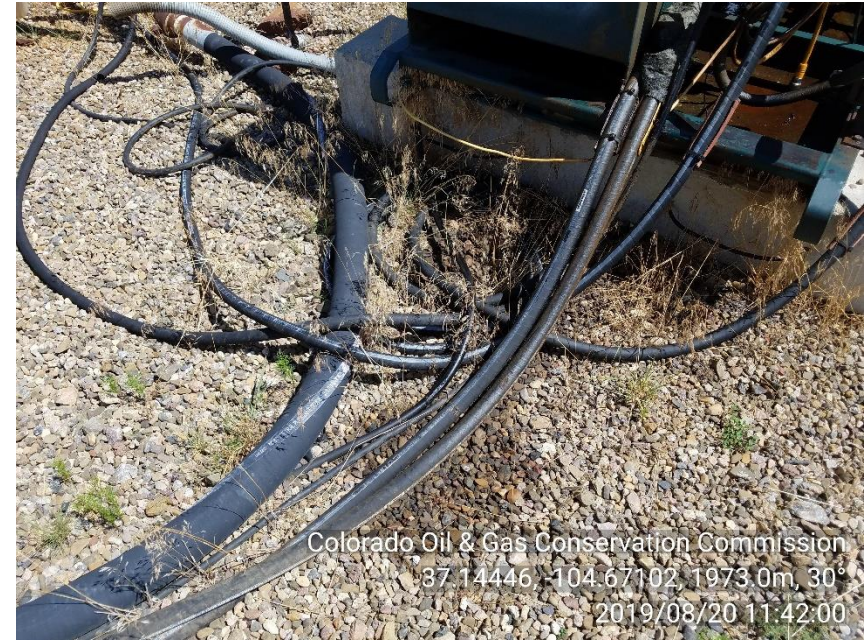
PHOTO 4: AREA OF IMPACTED SOIL NEAR HYDRAULIC CONNECTIONS ON DRIVEHEAD ENGINE SKID. Remove and dispose impacted material in approved manner, service and maintain equipment and self inspect to prevent recurrence of conditions per 1002.f(2) and 907. CA DATE 9/20/19.
