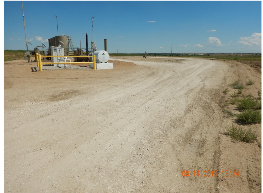
Photo 2. Photo taken from the entrance of the location, facing Southeast. Photo illustrates the Operator has reduced the size of the location only needed for production operations.
