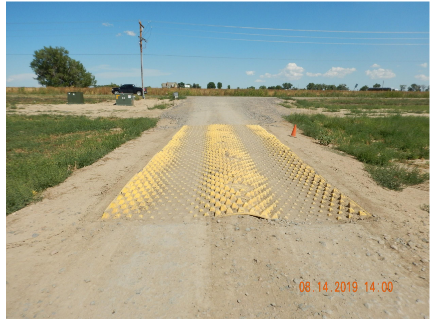
Photo 2. Photo taken from the entrance of the location, facing East. Photo illustrate the vehicle tracking device BMP is in need of maintenance and is not in proper functioning condition.
