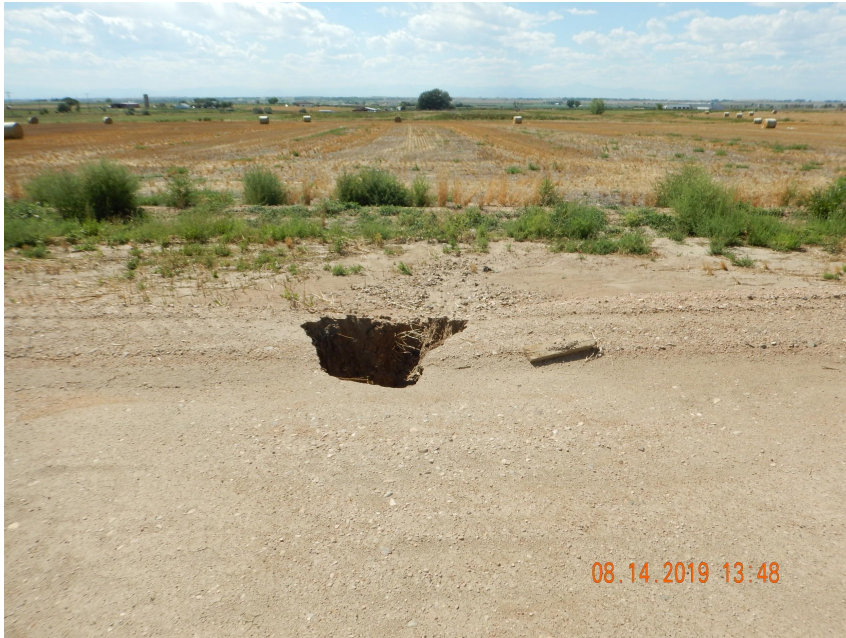
Photo 10. Photo taken from the western well pad, facing West. Photo illustrates erosion that has not been repaired.
