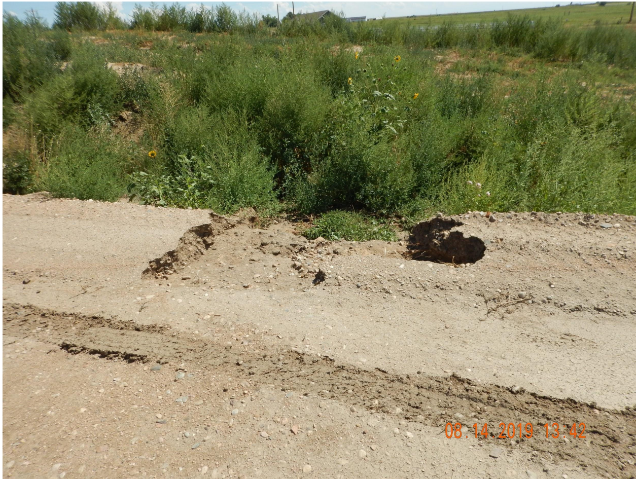
Photo 8. Photo taken from the southwestern well pad, facing South. Photo illustrates erosion that has not been repaired. Appears there was sediment discharge from location.
