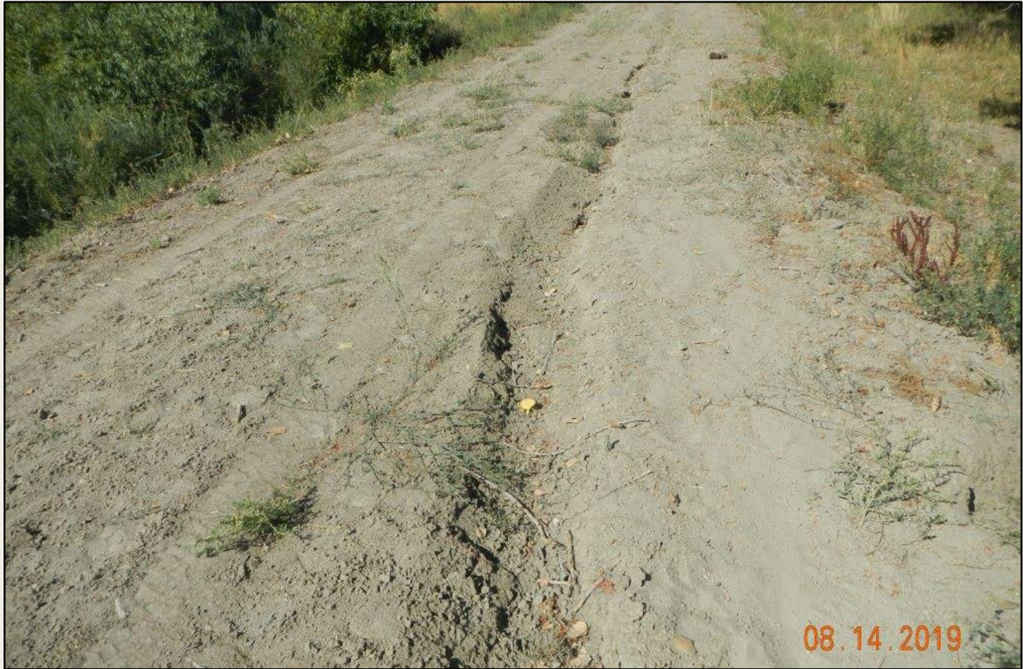
Photo 2. View of erosional channel forming within the access road slope.
