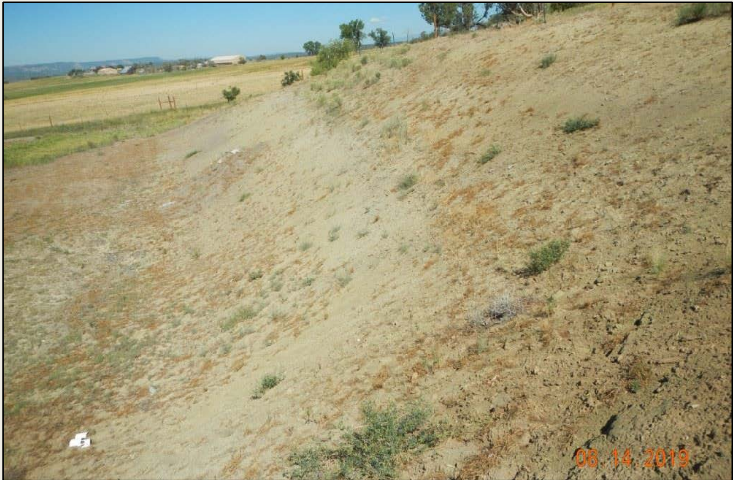
Photo 3. View of bare soils on the northern cut-slope.
