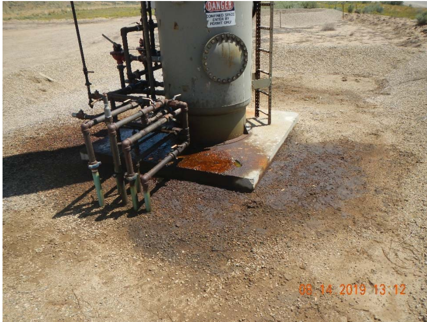
Photo 7. Stained soil and free fluid at separator.
