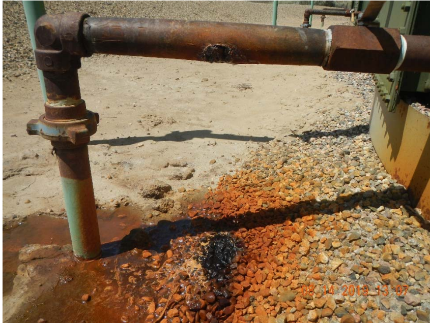
Photo 3. Ongoing leak occurring at tank flowline.
