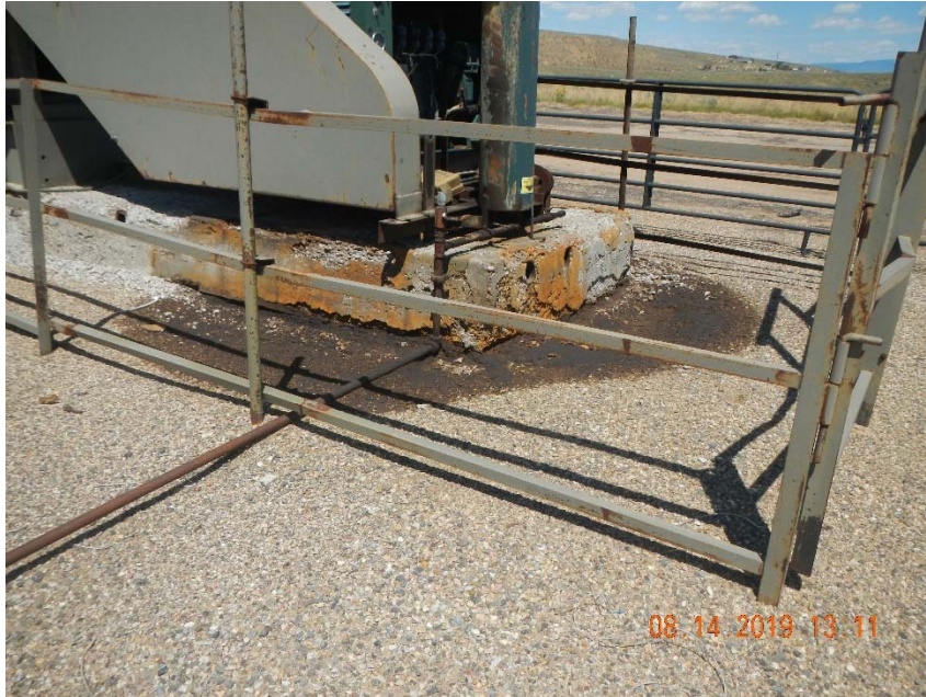
Photo 5. Stained soil at pump jack motor.
