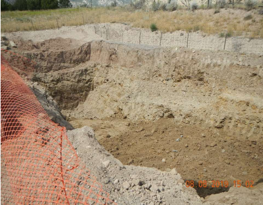
Photo #3 – View of the excavation looking north. The sidewalls of the excavation were moist but there was no hydrocarbon staining observed or odor.
