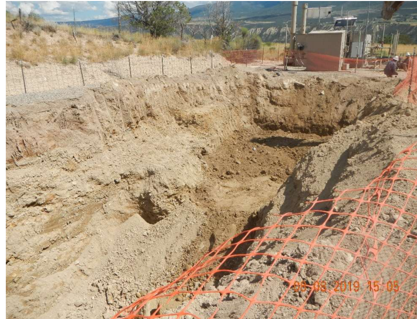
Photo #2 – View of the excavation looking south. The sidewalls of the excavation were moist but there was no hydrocarbon staining observed or odor.
