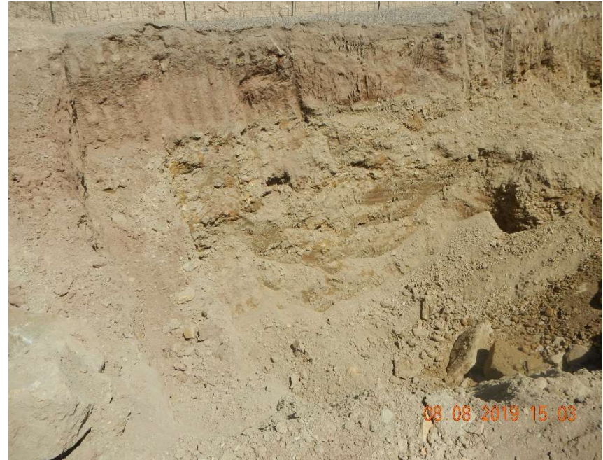
Photo #4 – View of the eastern excavation sidewall looking east. The sidewalls of the excavation were moist but there was no hydrocarbon staining observed or odor.
