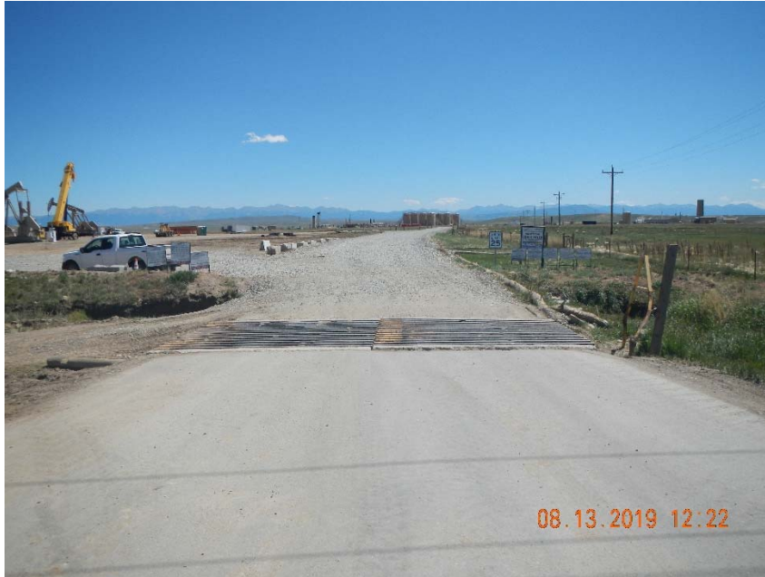
Photo 1. Rock added to area behind cattle guard. Tracking still occurring through cattle guard and onto concrete apron.
