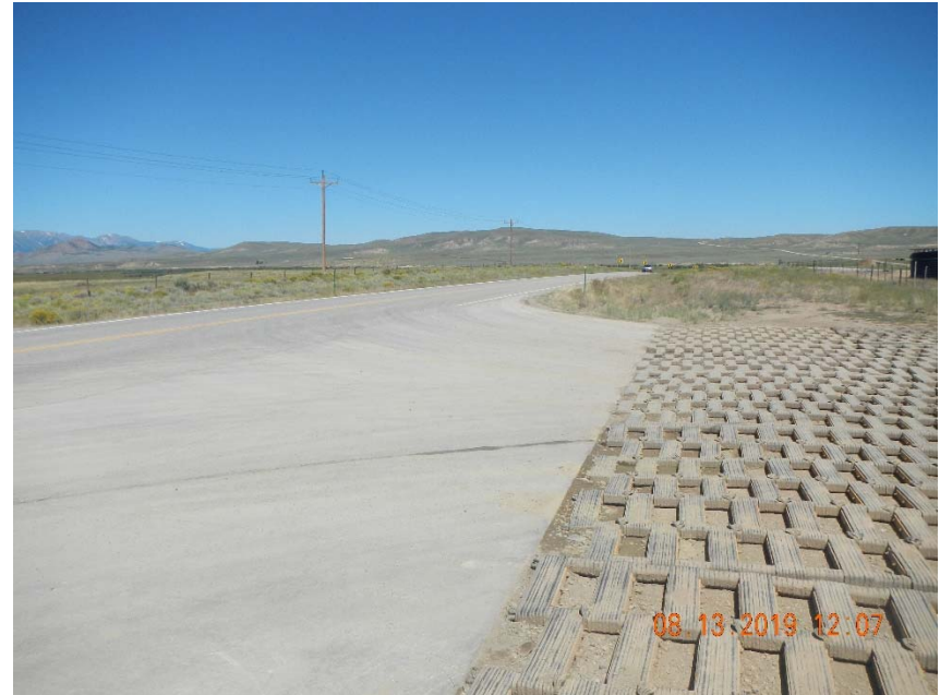
Photo 10. Tracking BMP on right side of photo, tracking onto highway 14 continuing to occur on left side of photo.
