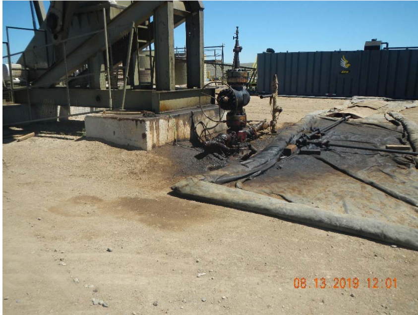
Photo 1. Non reportable spill at wellhead. Containment that has become trash/debris at wellhead.
