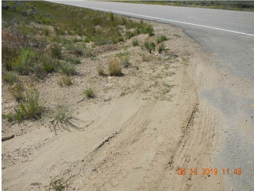
Photo 7. Sediment migrating off location and into ditch. 8/13/2019
