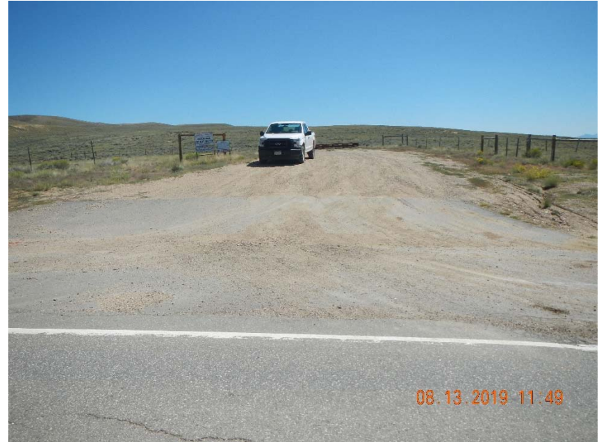
Photo 6. Tracking onto highway 14. 8/13/2019
