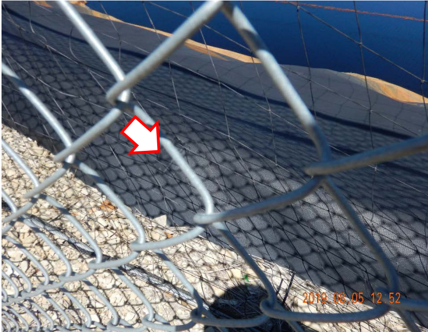
Photo #5 – Liner patch in southern portion of east berm.
