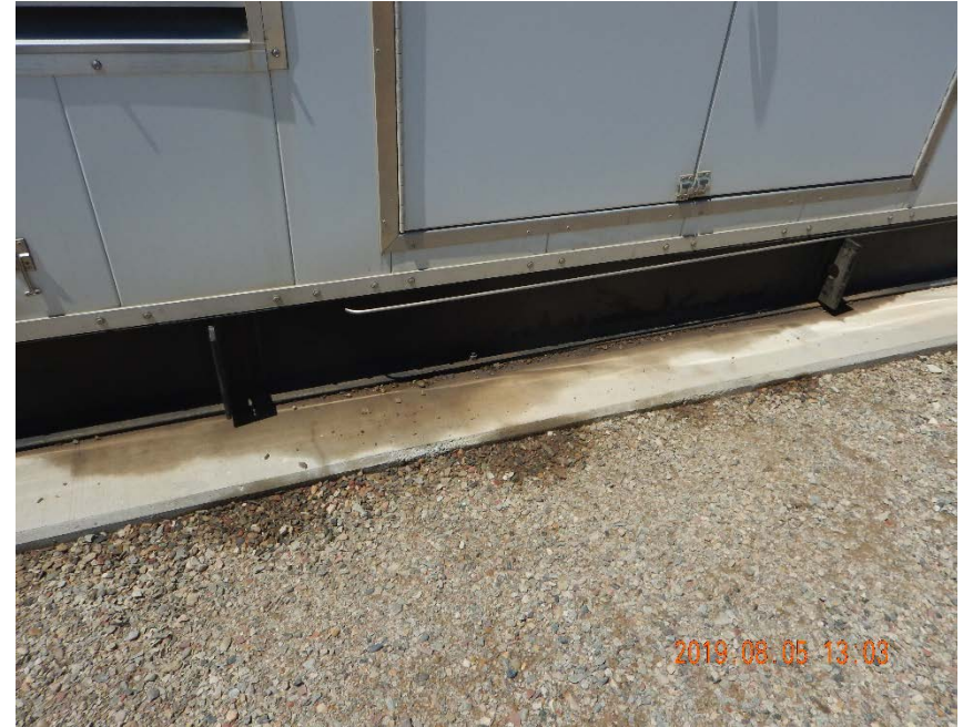
Photo #14 – Localized accumulations of stained gravel and possible staining observed on top of east side of concrete pad beneath compressor shed located north of Cascade Creek #616-21-32 (API #045-10444) well.
