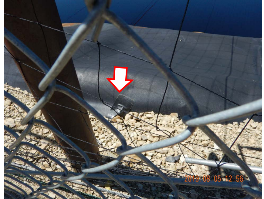
Photo #6 - Liner patch in southern portion of east anchor trench.
