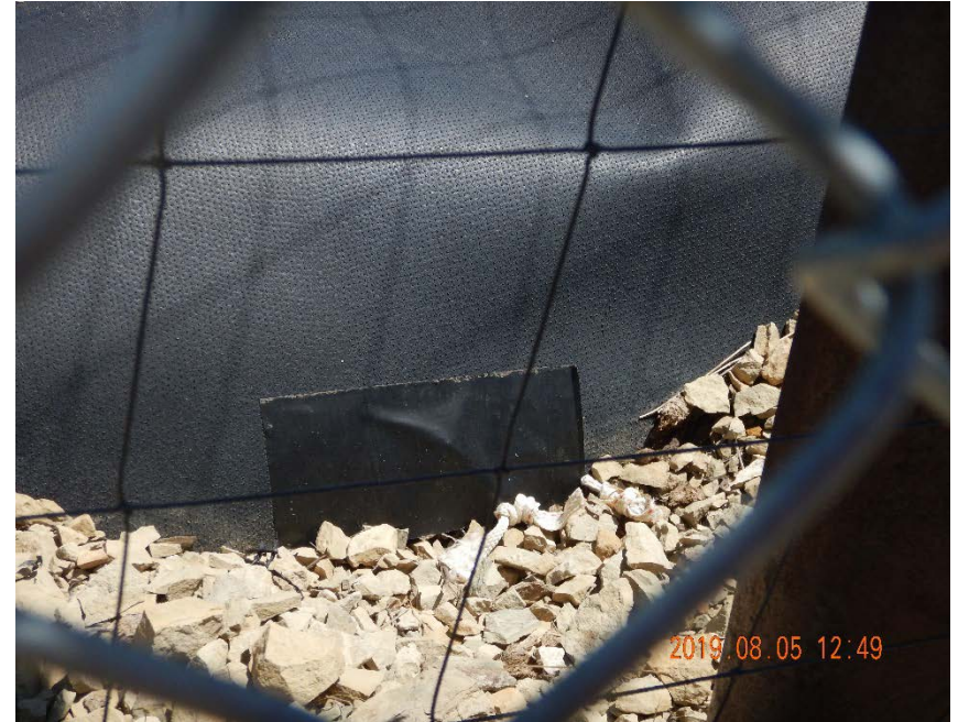
Photo #2 – Liner patch in southern portion of west anchor trench.
