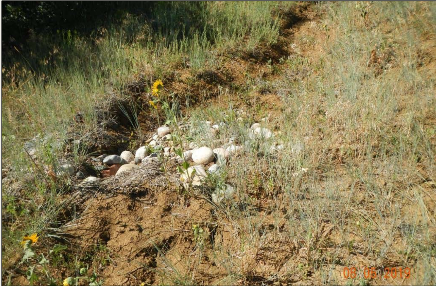
Photo 2. View of BMP that is not sufficient and erosion is continuing within the southeastern project area.
