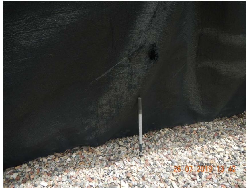
Photo #4 – Hole in liner.
