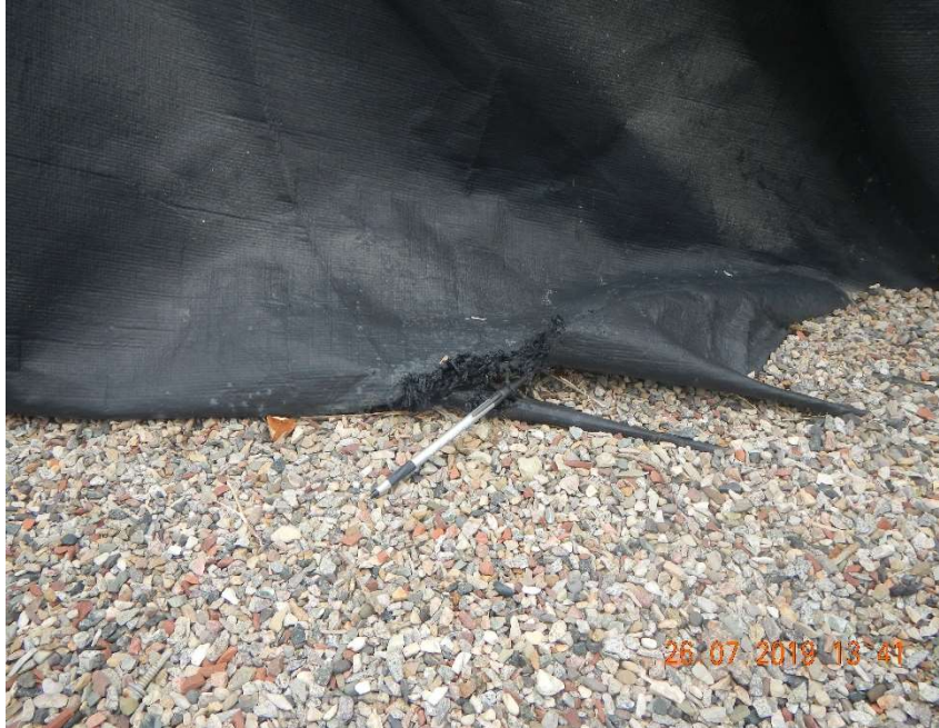
Photo #5 – Hole in liner.
