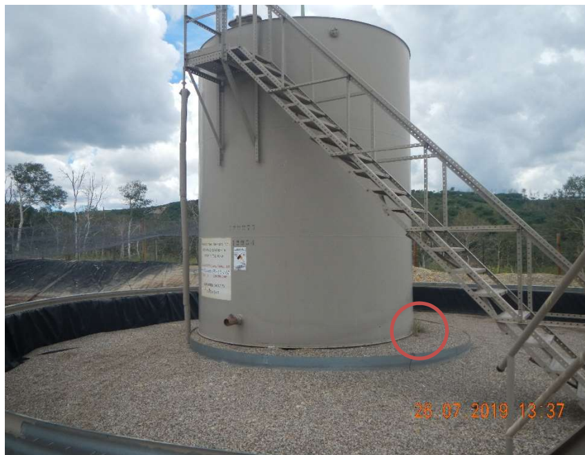
Photo #7 – Vegetation within secondary containment.
