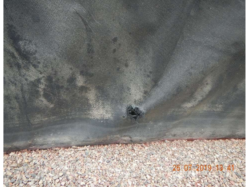
Photo #6 – Hole in liner.
