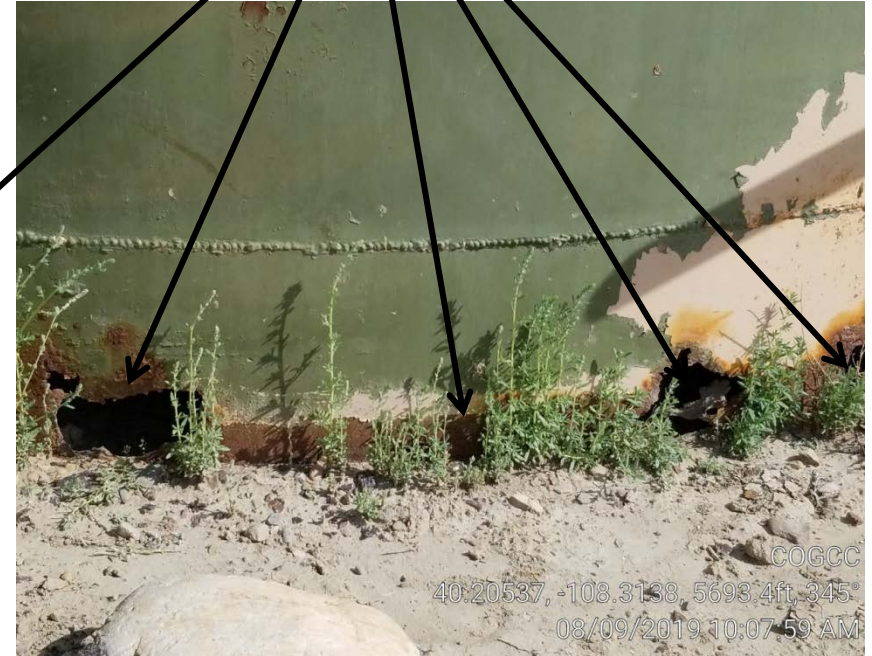
Photo 7. Unused tank holes.
