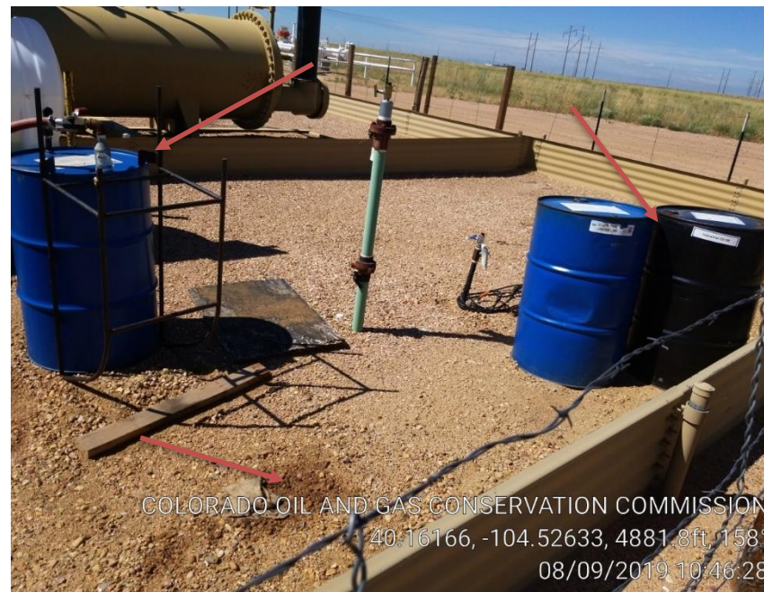
Pic 6 unused equipment/trash/no containment on chemical tanks/stained soil
