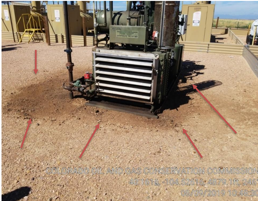
Pic 9 stained soil/mechanical issues/spill
