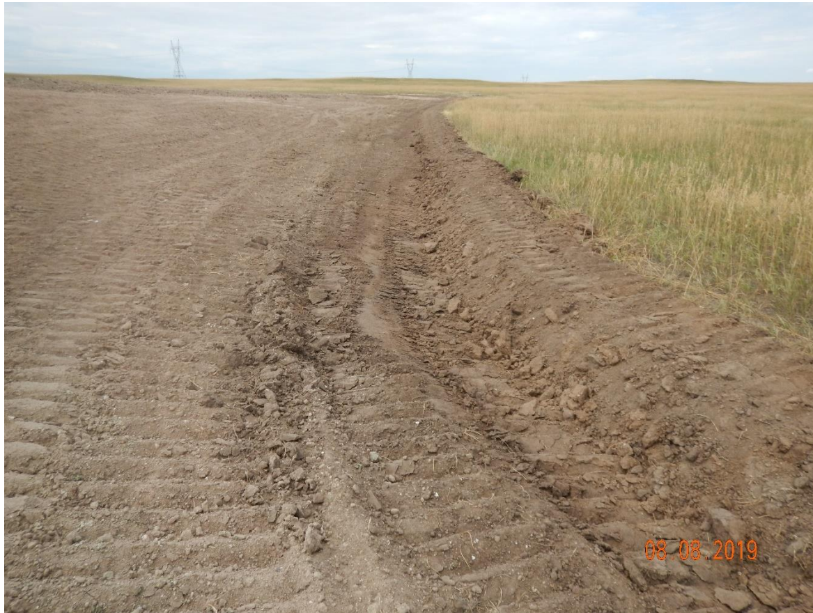
Photo 11: Photo taken from the north end of the location, facing west. Photo shows tracking on slopes and perimeter stormwater diversion ditch/berm have not been installed in accordance with good engineering practices. See comments under photos 5 and 7.
