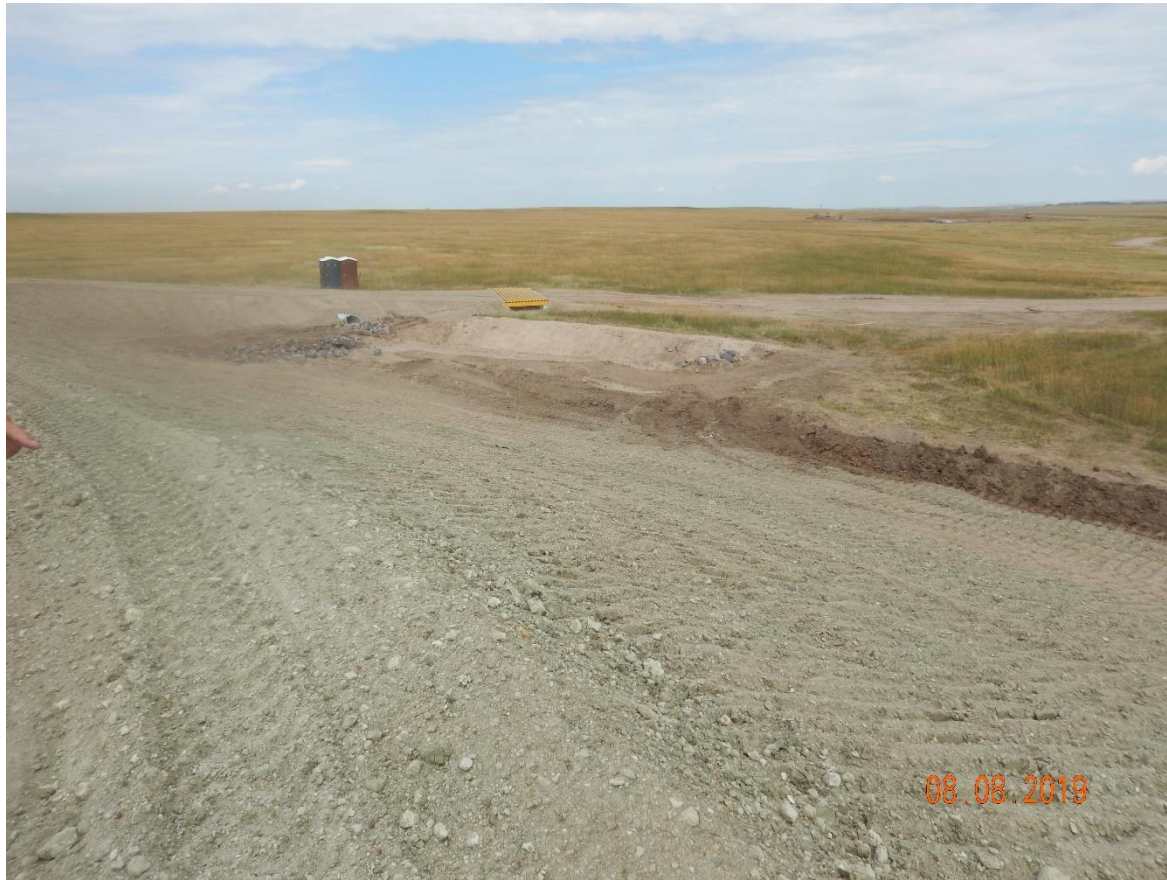
Photo 8: Photo taken from north end of the pad, facing north. Photo shows one of the three sediment traps along the perimeter of the location. Traps appear to be sufficient in size, however, sediment traps have not been constructed in accordance with good engineering practices; Berms and slopes at traps remain unconsolidated. BMPs missing inlet armoring/protection. Rock aggregate used for outlet protection appears too large in size to slow stormwater discharge, trap sediment and sufficiently stabilize outlet.
