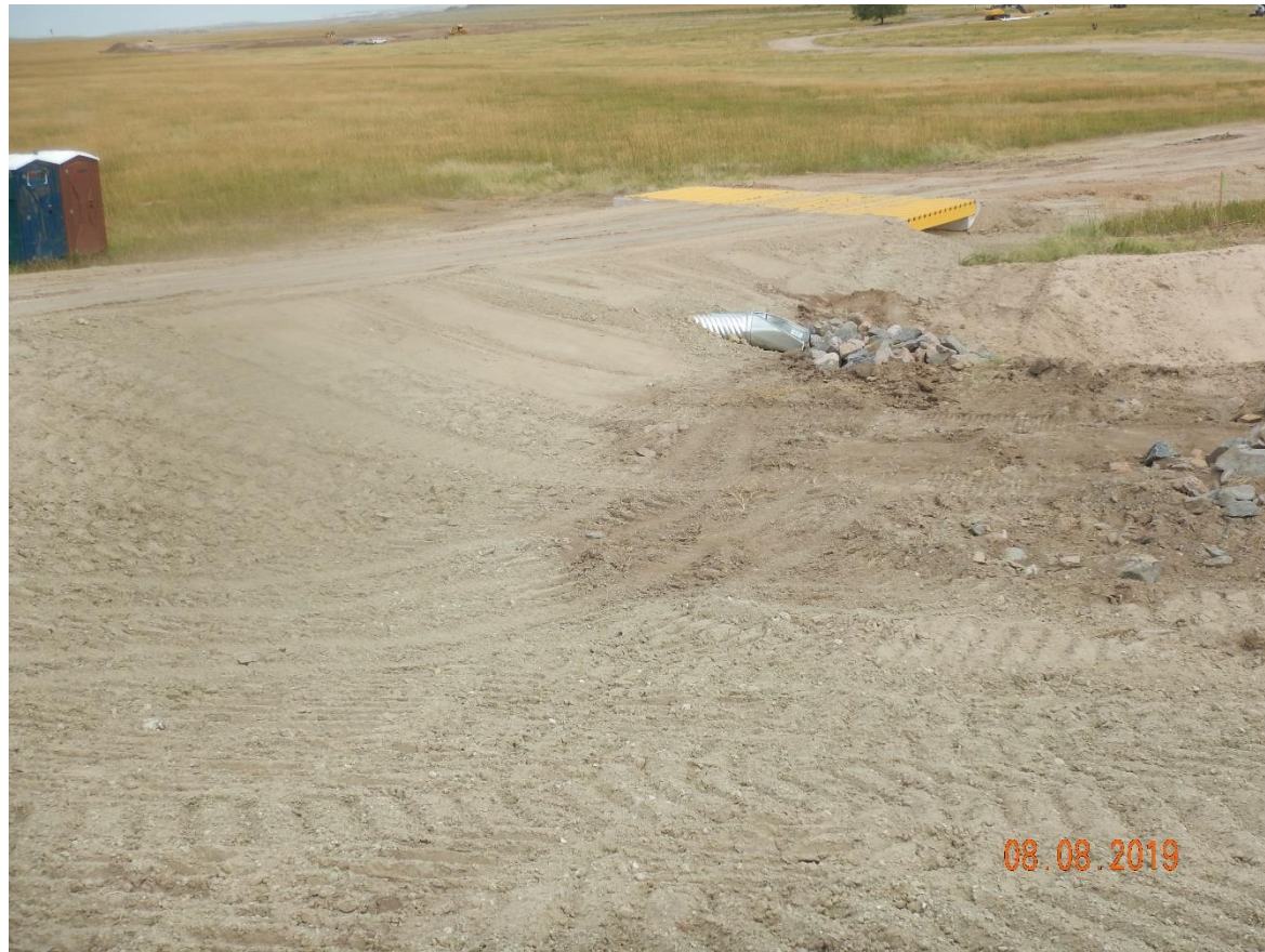
Photo 10: Photo taken from the north end of the location. Photo shows insufficient armoring/stormwater protection at culvert.
