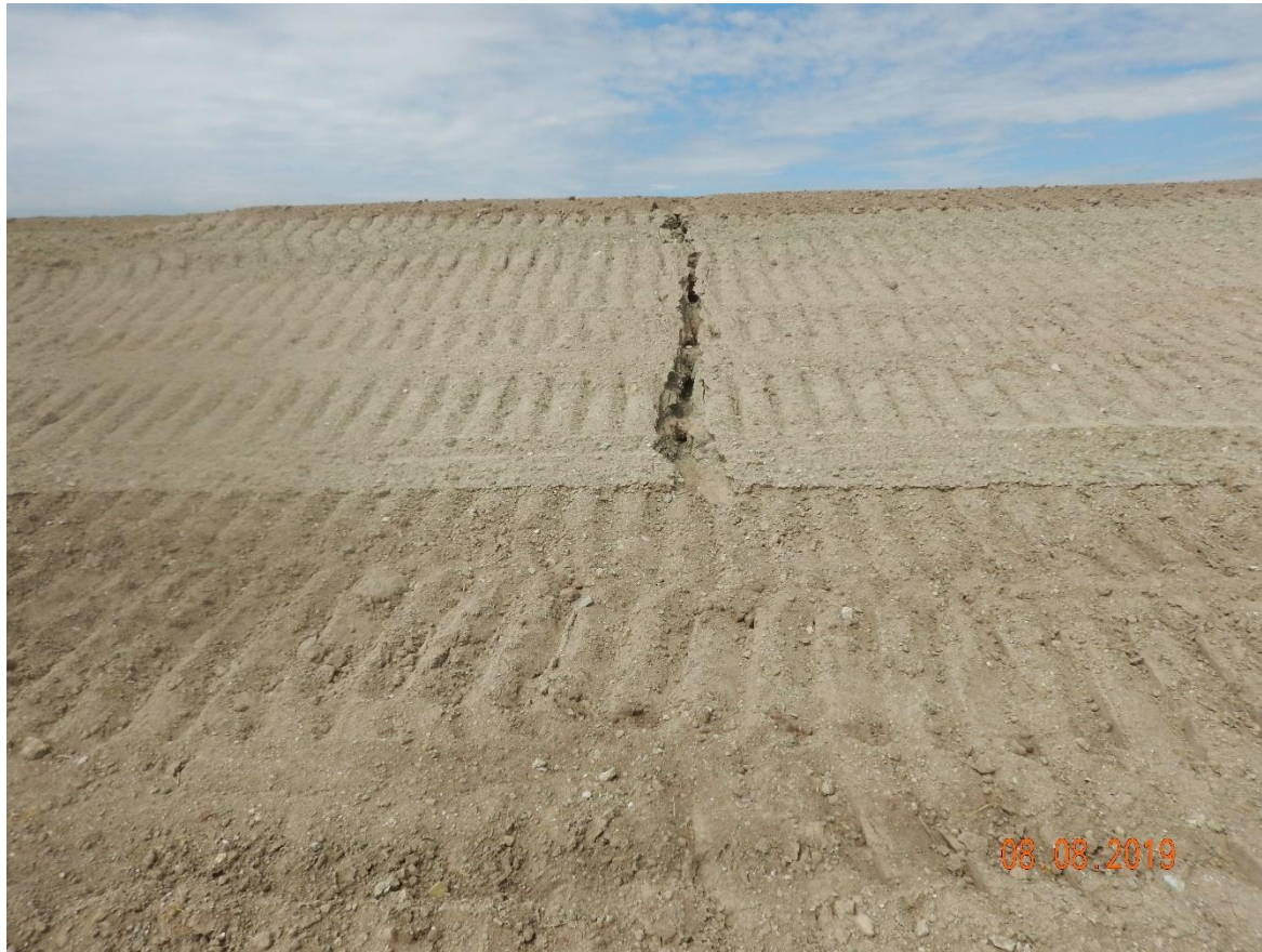
Photo 5: Photo taken from the slopes on the east end of the location. Photo shows operator has installed tracking BMP to stabilize the slopes on the location. BMP has not been installed in accordance with good engineering practices. Tracking has not been installed up and down the slope, thus facilitating gulley erosion degradation.
