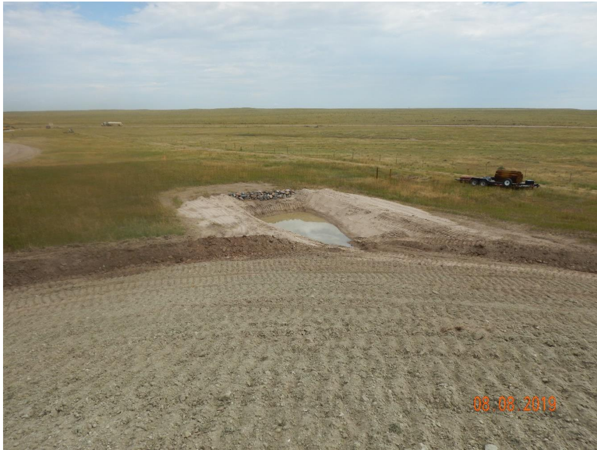
Photo 9: Photo taken from north end of the pad, facing northeast. Photo shows one of the three sediment traps along the perimeter of the location. See comments under photo 8.
