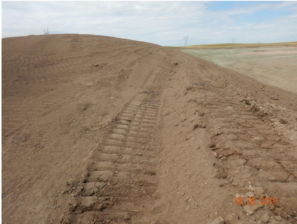
Photo 7: Photo taken from the topsoil stockpile on the south end of the location. Three stormwater diversion ditch/berms have been constructed: 1 @ the pad perimeter, 1@ base of the soil stockpiles, and 1@ the perimeter of the disturbance area. Ditch/berm have not been installed in accordance with good engineering practices; Ditch/berm remains loose, unconsolidated material, that will contribute to sediment laden stormwater discharge. Photo also shows tracking on slopes is insufficient (See photo 5)
