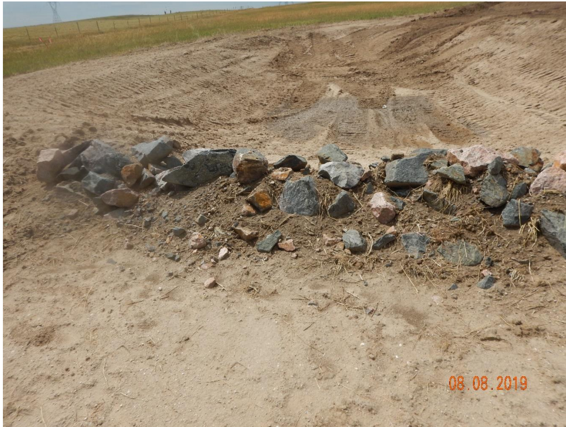
Photo 6: Photo taken from the southeast end of the location. Photo shows one of the three stormwater sediment traps on the location. Traps appear to be sufficient in size, however, sediment traps have not been constructed in accordance with good engineering practices; slopes at traps remain improperly tracked. BMPs missing inlet armoring/protection. Rock aggregate used for outlet protection appears too large in size to slow stormwater discharge, trap sediment and sufficiently stabilize outlet. Additionally outlet has been intentionally filled with material. This forces outlet to work as a dam, rather than allowing for sediment laden free stormwater discharge.
