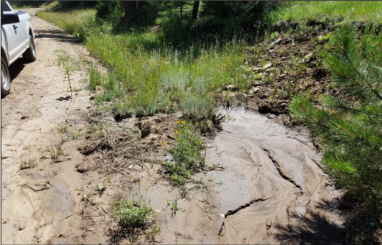
Photo 3. The culvert has filled in with sediment along the main road.
