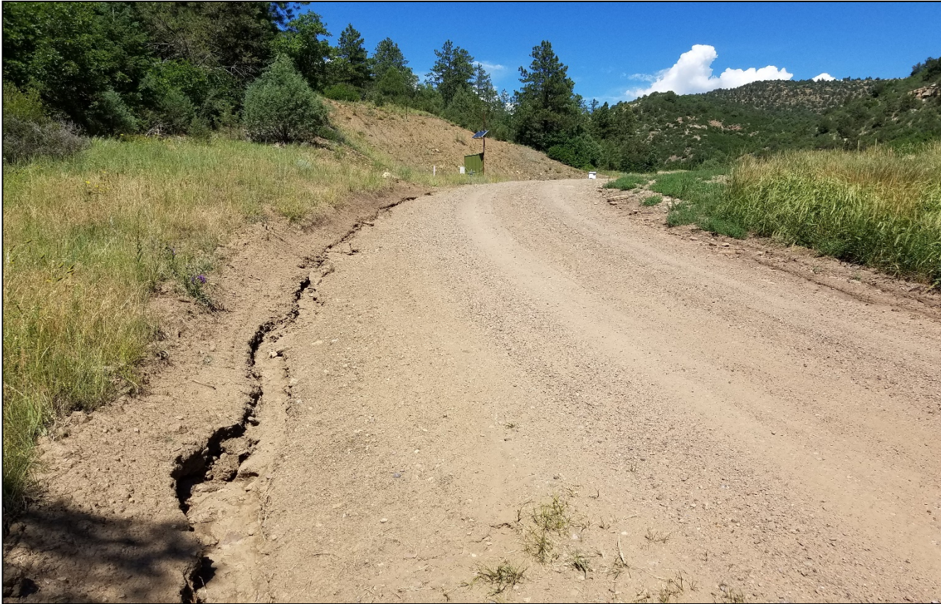
Photo 5. Erosion channel has already developed where erosion was repaired. BMP's need to be installed to control erosion.
