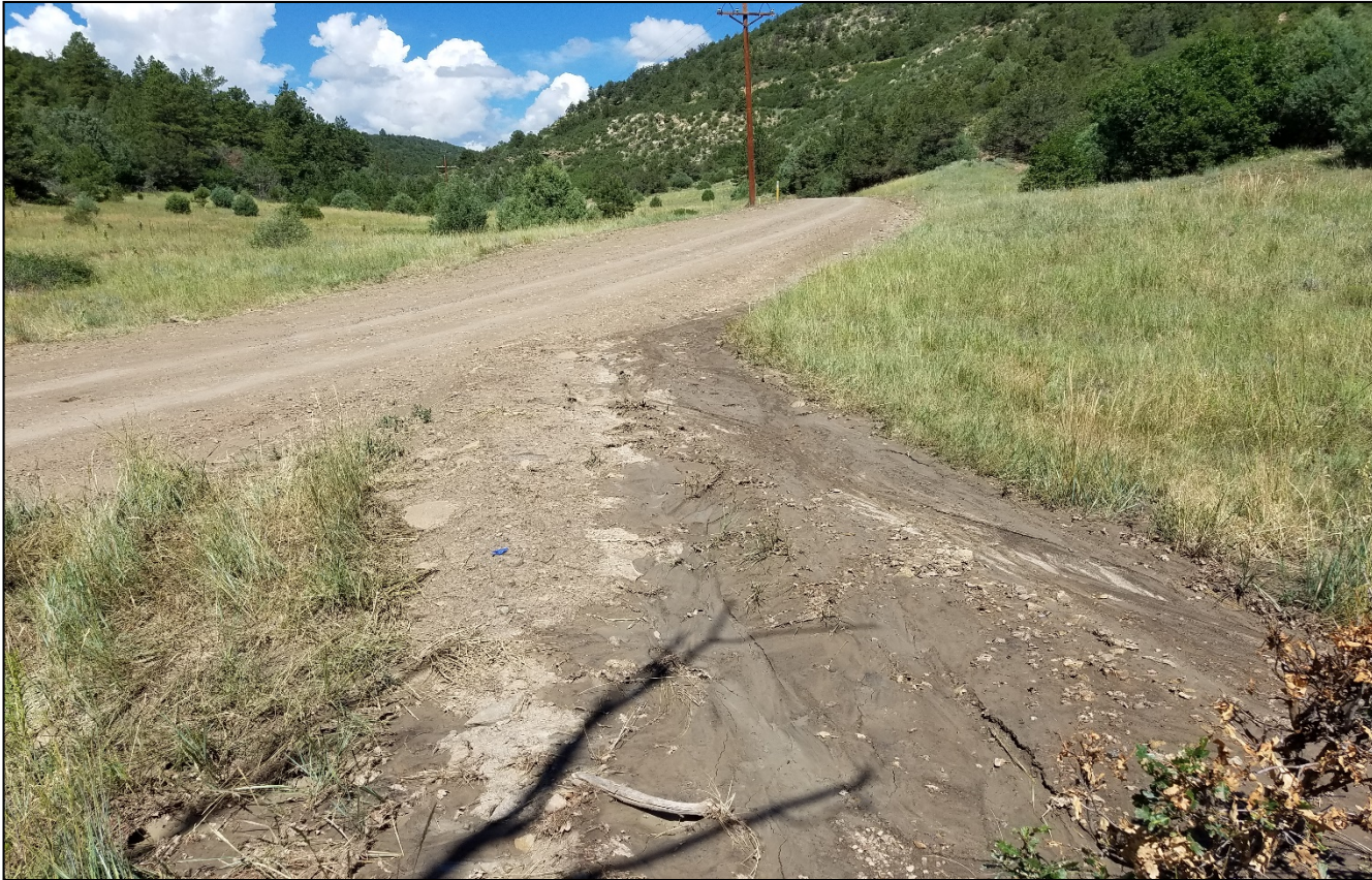
Photo 2. Sediment has already filled into the diversion ditch since grading occurred. A sediment trap or rock checkdamns may be need to control erosion.
