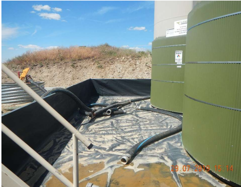
Photo #9 - Assorted metal equipment stored in direct contact with tank battery liner.
