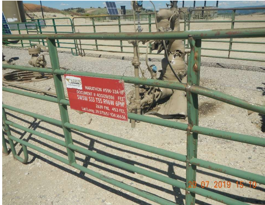
Photo #5 - Localized accumulation of oily waste (oil-stained soil) in the 596-33C-18 cellar.
