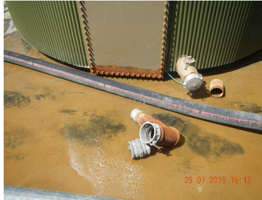
Photo #10 - Assorted metal equipment stored in direct contact with tank battery liner.
