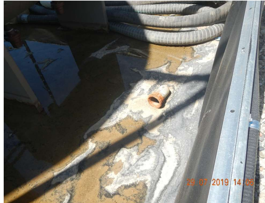
Photo #6 – Metal equipment stored directly on liner.
