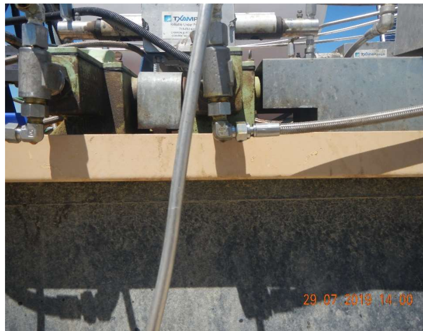
Photo #4 – View of active leak at the process pipe pump control area.
