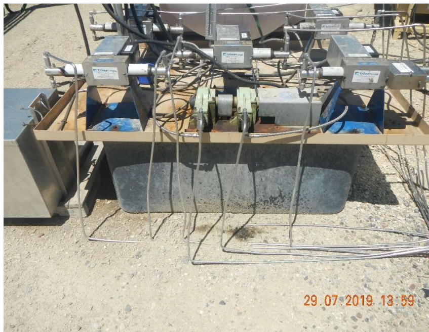
Photo #3 – View of active leak at the process pipe pump control area.
