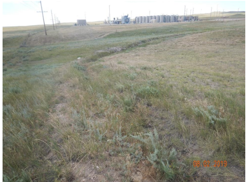
Photo 8: Photo taken from the south end of the location, facing west. Photo shows the perimeter stormwater ditch during initial construction activities remaining. Vegetation over interim areas appear to have sufficiently stabilized the soils; Original perimeter stormwater ditch, sediment traps, BMPs etc... no longer appear to be necessary and require reclamation..
