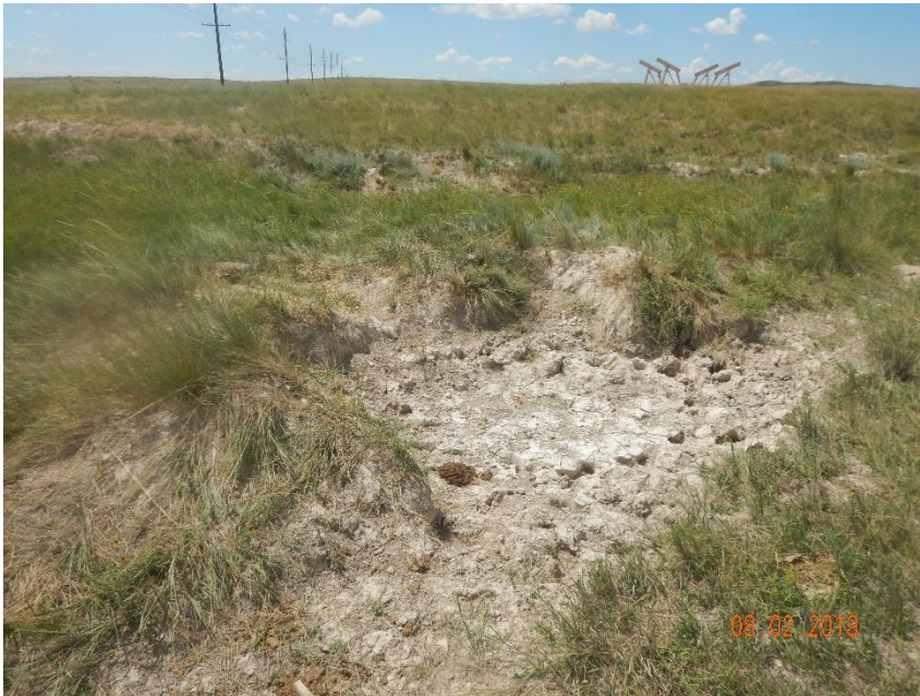
Photo 13: Photo taken from the southwest end of the location, facing west. Photo shows the perimeter stormwater ditch and sediment trap BMPs during initial construction activities remaining. BMPs have not been maintained, do not appear to be needed and require reclamation.
