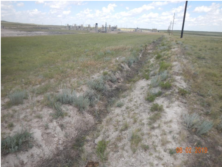
Photo 11: Photo taken from the south end of the location, facing east. Photo shows the perimeter stormwater ditch during initial construction activities remaining. BMPs have not been maintained, do not appear to be needed and require reclamation.
