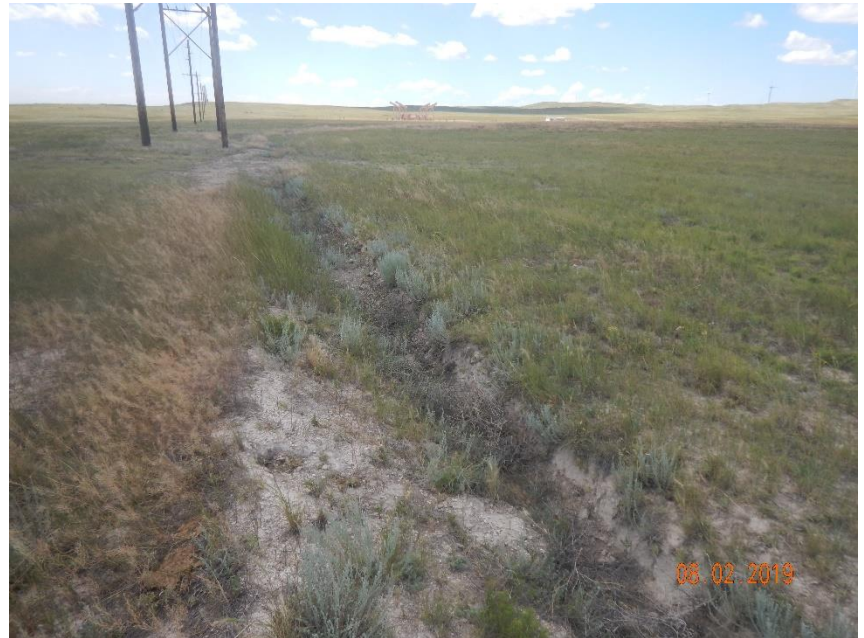
Photo 10: Photo taken from the south end of the location, facing west. Photo shows the perimeter stormwater ditch during initial construction activities remaining. BMPs have not been maintained, do not appear to be needed and require reclamation.
