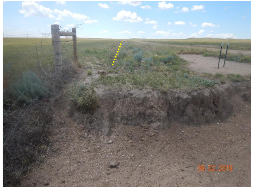
Photo 14: Photo taken from the north end of the location, facing west. Photo shows the perimeter stormwater ditch during initial construction activities remaining. BMPs have not been maintained, do not appear to be needed and require reclamation.
