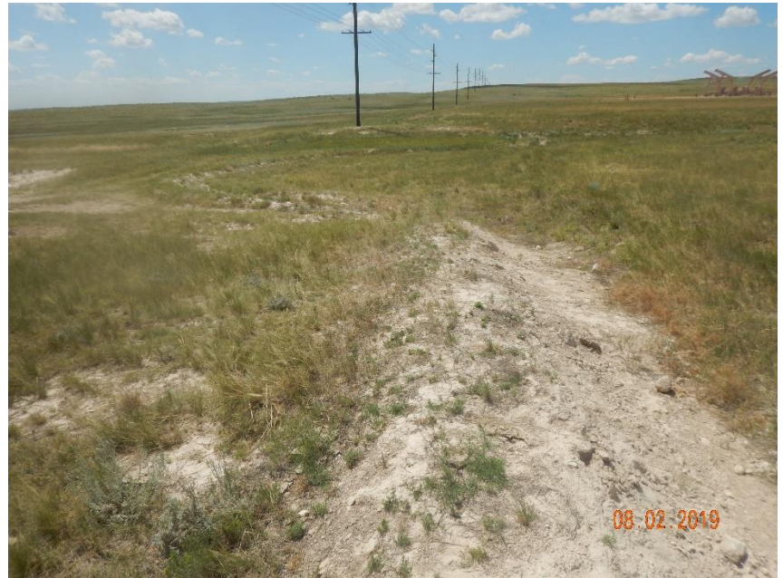
Photo 12: Photo taken from the southwest end of the location, facing west. Photo shows the perimeter stormwater ditch during initial construction activities remaining. BMPs have not been maintained, do not appear to be needed and require reclamation.
